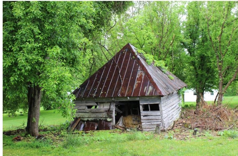
Smoke house (one of two remaining original structures)
