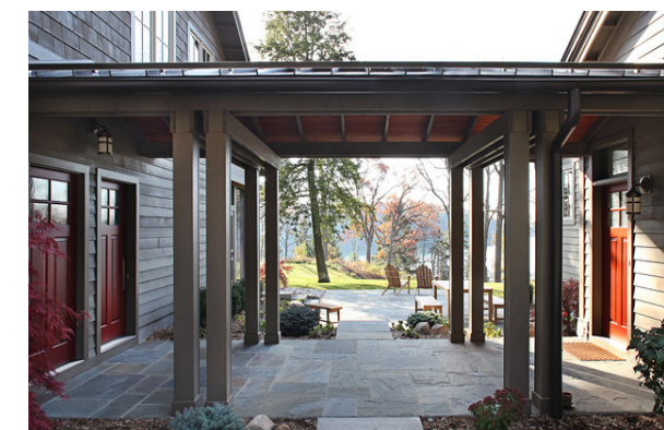
Breezeway between Barns
