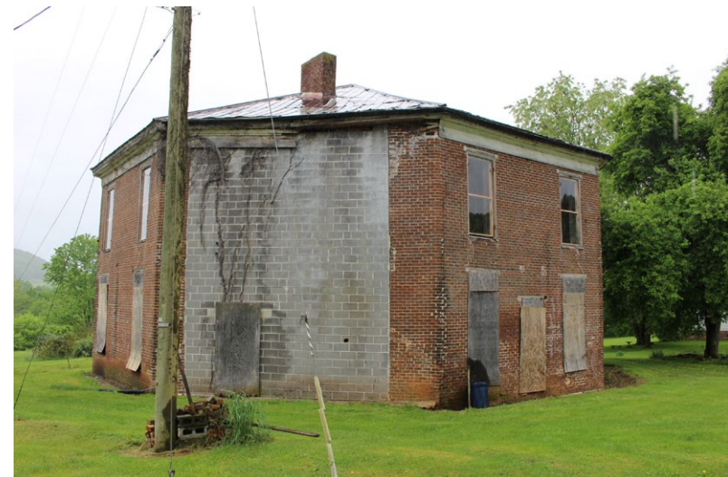
The approximate location of the underground historic cistern on the right.
