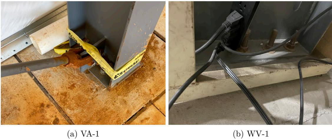
Figure 4.53: Close up view of the column bases for two different metal buildings
