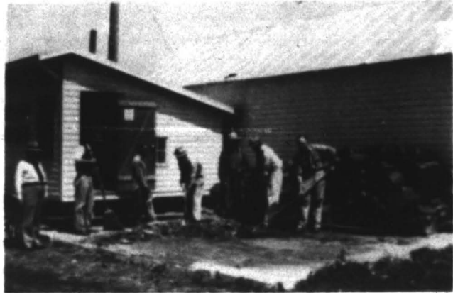
When brooder houses cannot be moved to clean ground, a concrete runway will help keep down diseases and parasites.
