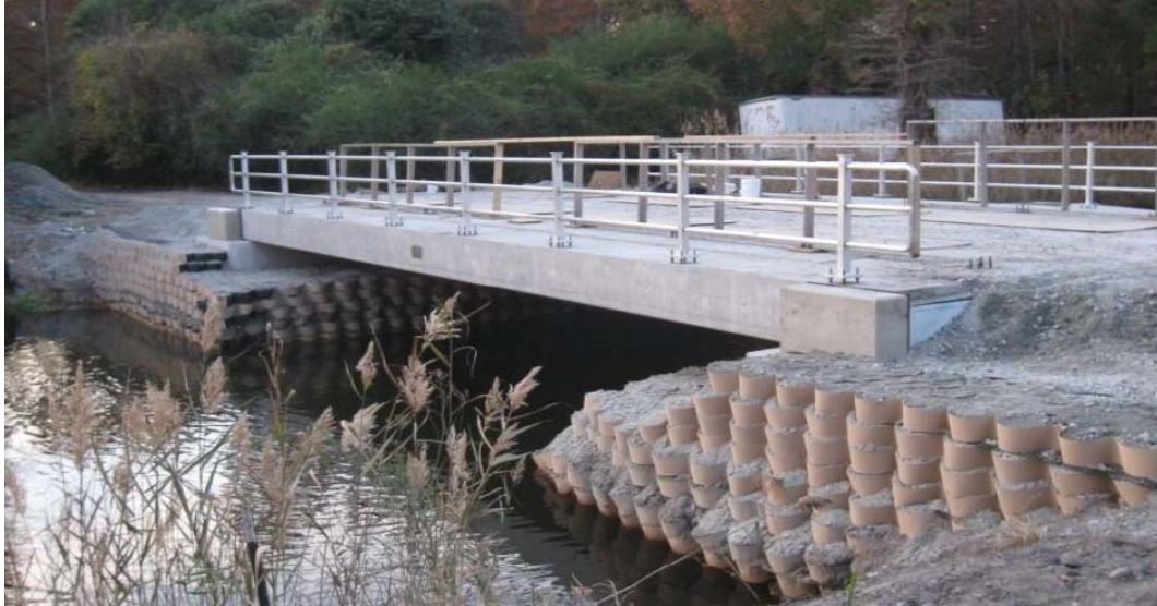
Figure 12: Mattamuskeet National Wildlife Refuge GRS Bridge Nguyen, Q. (2012). "GRS Abutments for Bridge Replacement National Wildlife Refuge." A New Era of Partnerships - Investing in America's Treasures, U.S. Department of Transportation, FHWA, EFLHD. Used under fair use, 2014.
