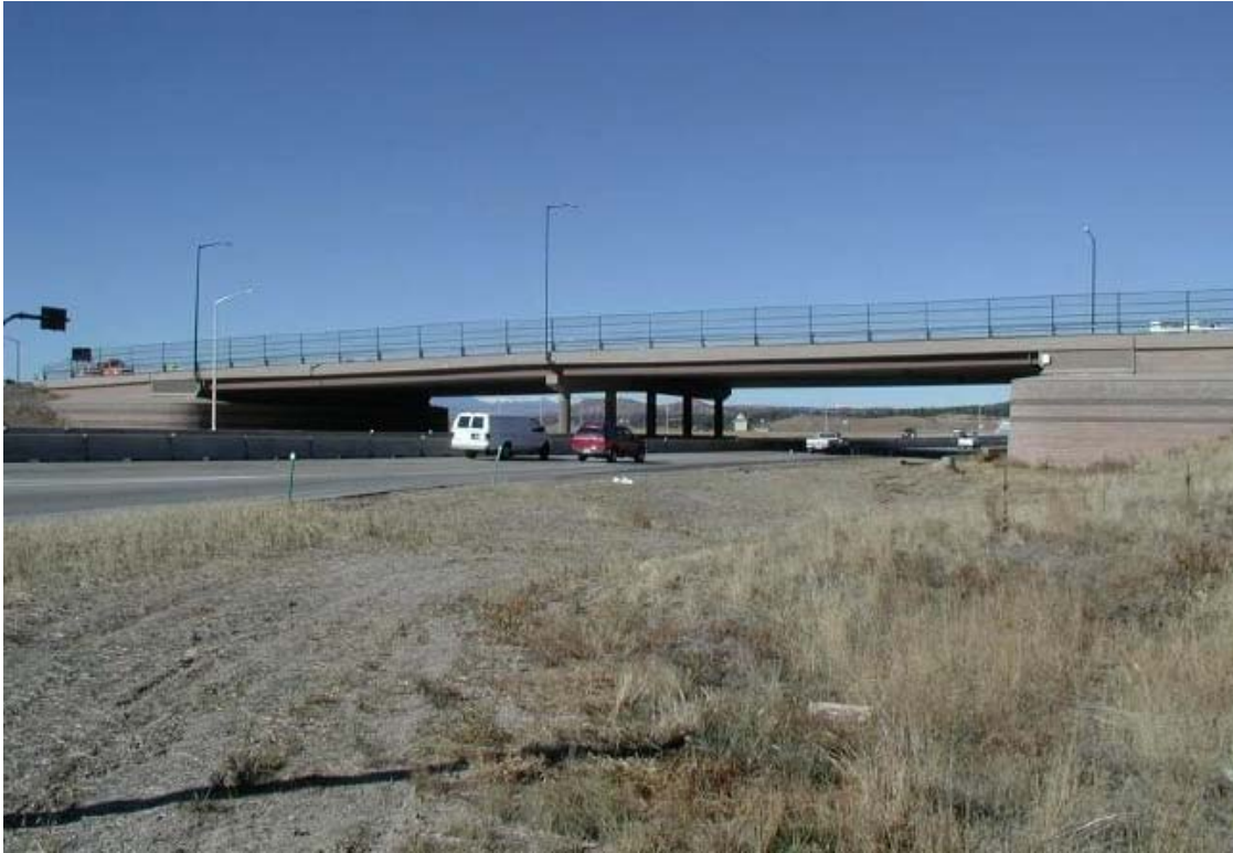
Figure 7: Founders/Meadows Parkway Structure Wang, T. (2002). "Case History of GRS Abutment." Workshop on Geotechnical Composite Systems, Sponsored by National Science Foundation and Virginia Tech, Roanoke, VA. Used under fair use, 2014.
