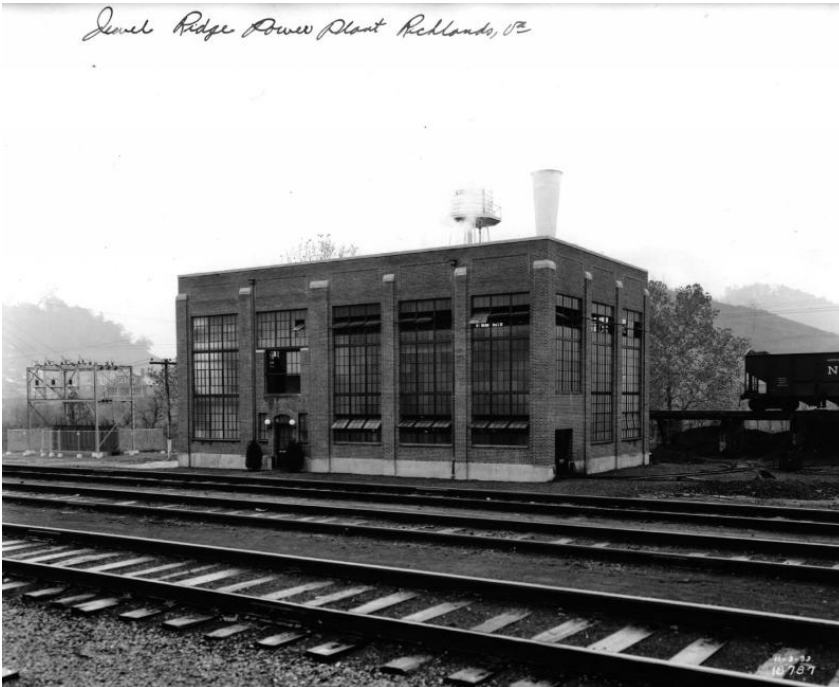
Jewell Ridge Power Plant, Jewell Ridge, VA (Library of Virginia)
