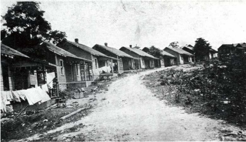
PORTION OF THE EAST END OF MAIN STREET JEWELL RIDGE COAL CORPORATION, JEWELL RIDGE, VA.
