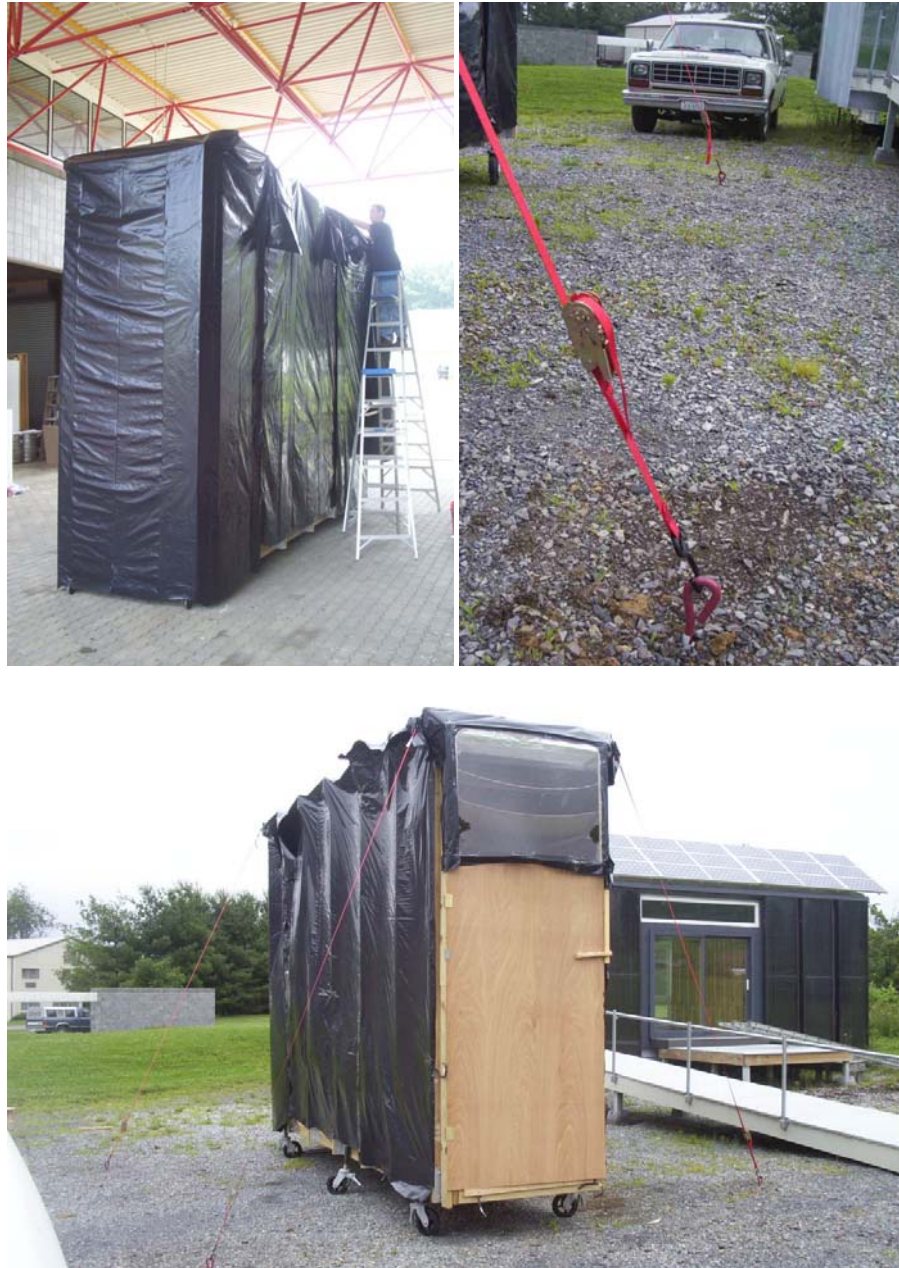
Figure 3.17: The arrangement for rain protection and wind force resistance
