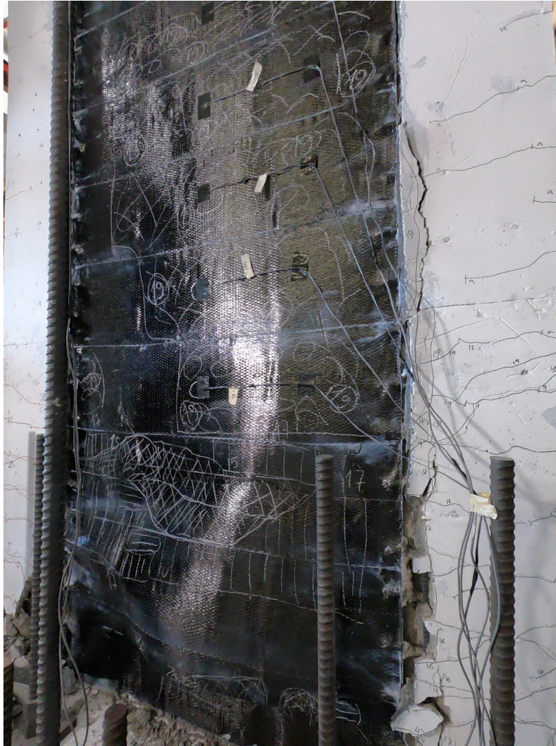
Figure 4.20: Final Damage State of S1FW - Anchor Pullout and Pilaster Vertical Crack
