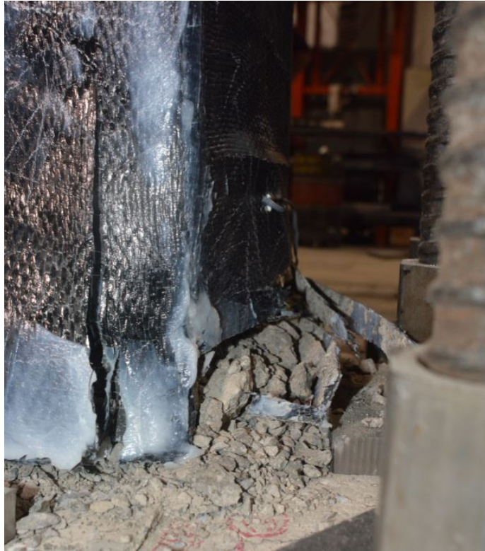
Figure 4.32: South Pilaster- Final Condition of Specimen S1FP
