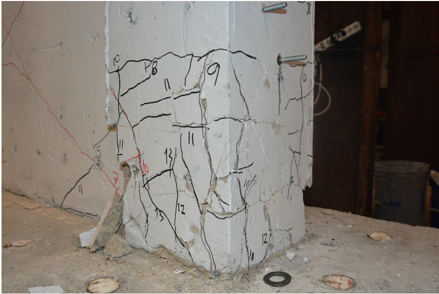
Figure 4.42: Lap Splice Region of Specimen S2- Final Condition
