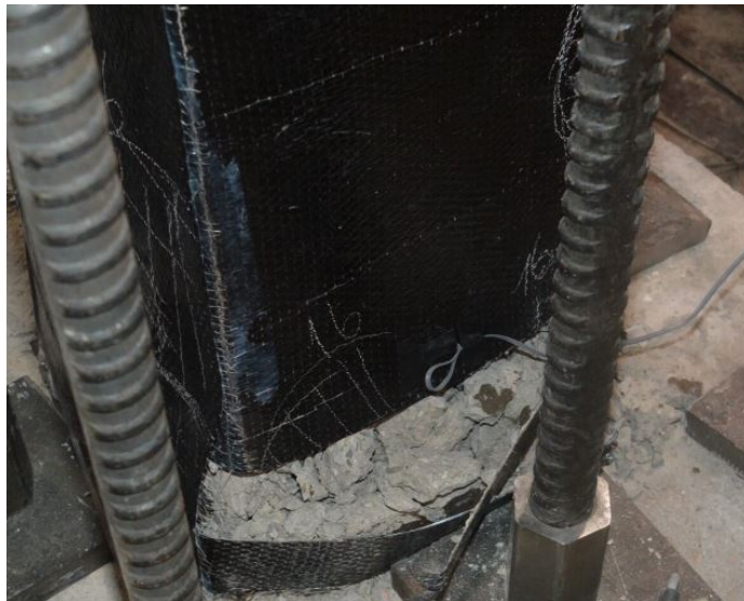
Figure 4.33: North Pilaster- Final Condition of Specimen S1FP
