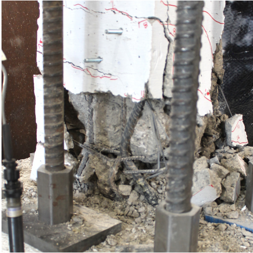
Figure 4.22: South Toe of Specimen S1FW Final State Photo - Bar buckling
