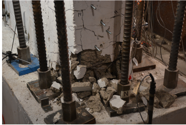
Figure 4.14: North Toe Final State of Specimen S1CW - Bar Buckling
