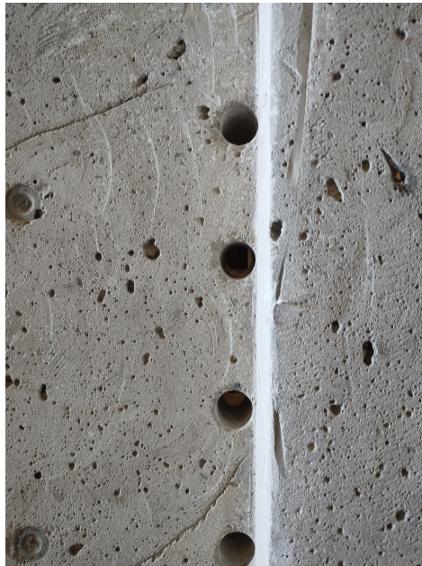
Figure 3.11: FRP Surface Preparation Photo
