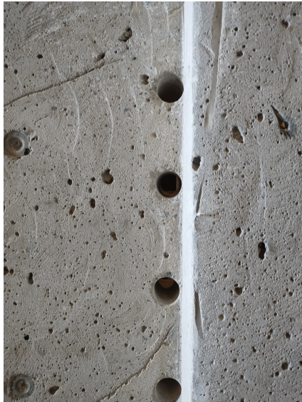
(a) Surface Preparation and Anchor Holes
