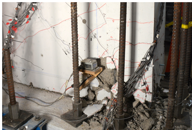
Figure 4.13: Web Crushing of Specimen S1CW
