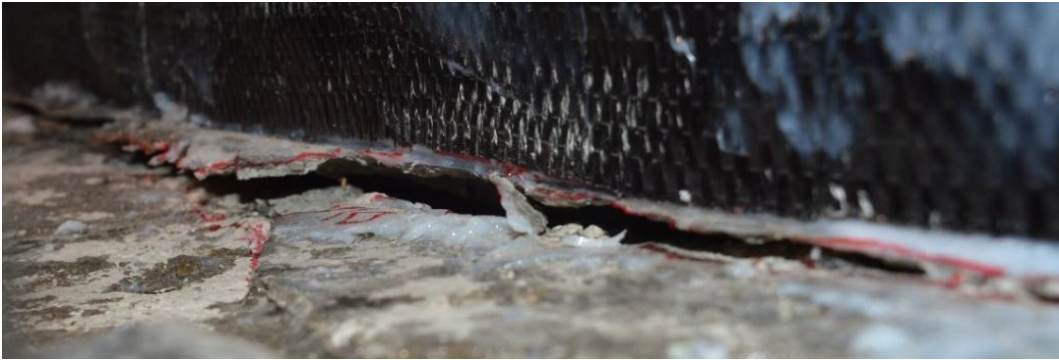
Figure 4.46: Close up of Final Base Crack of Specimen S2FL
