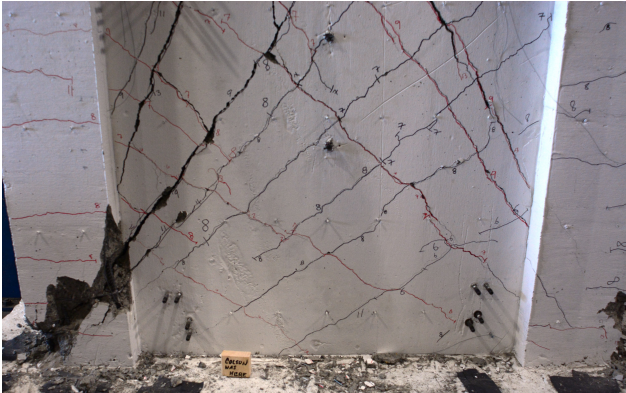
Figure 4.6: S1 Final Lower Wall Close Up
