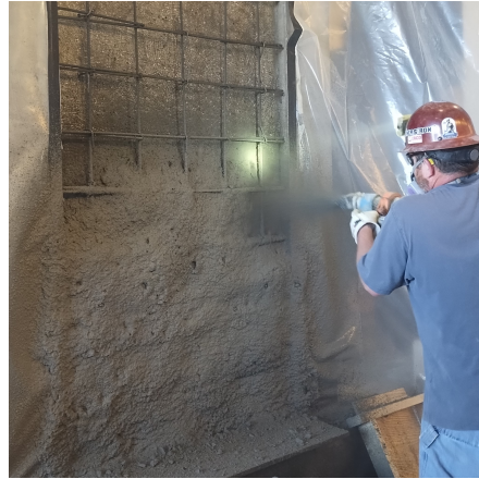
Figure 2.3: Shotcrete Installation
