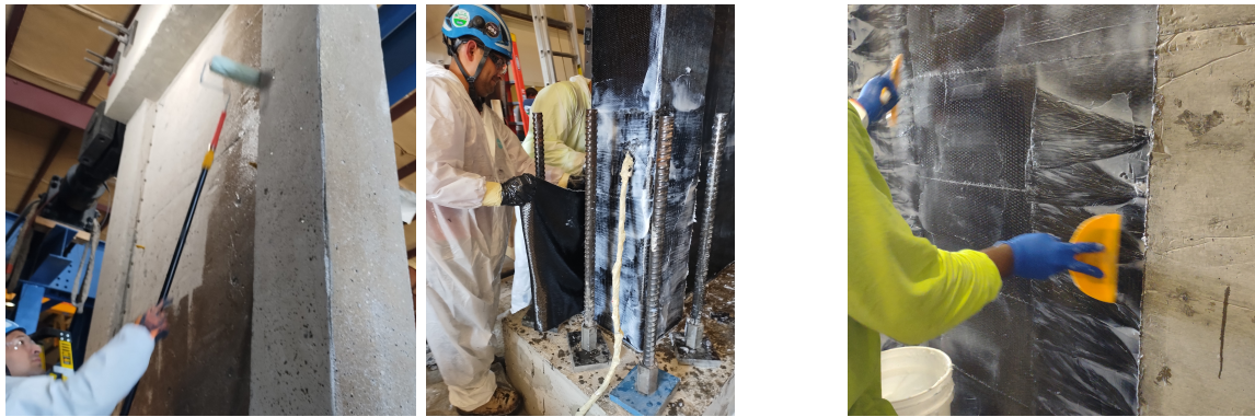
(a) Initial Epoxy Coat
