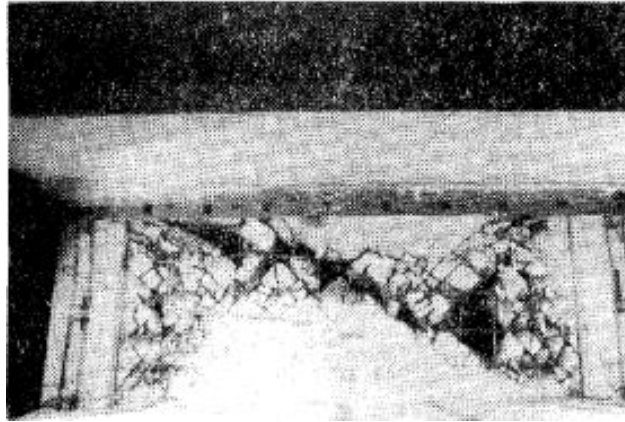
Figure 2.8: Experimental Specimen Web Damage from Iliya and Bertero (1980)
