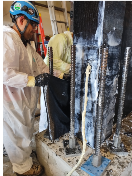
(b) FRP Sheet Installation
