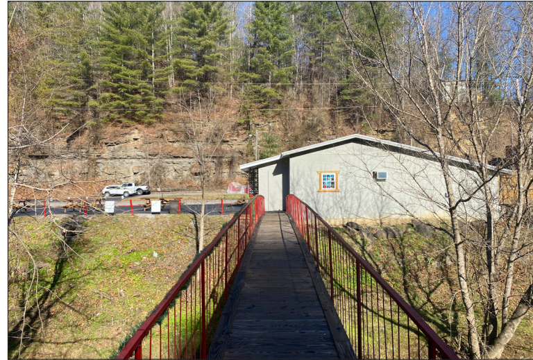
View of Historical Society of the Pound Bridge facing northeast, crossing Pound River to the Historical Society of the Pound.
