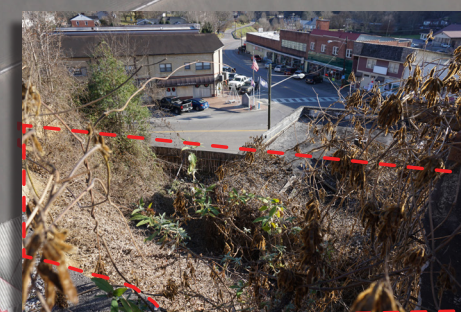
D. View of future trailhead location, roughly 40 feet above site on Church Street. The site's steep back-slope will need retaining wall. Site is currently inaccessible but this viewshed shows the future trailhead's location in downtown Pound.
