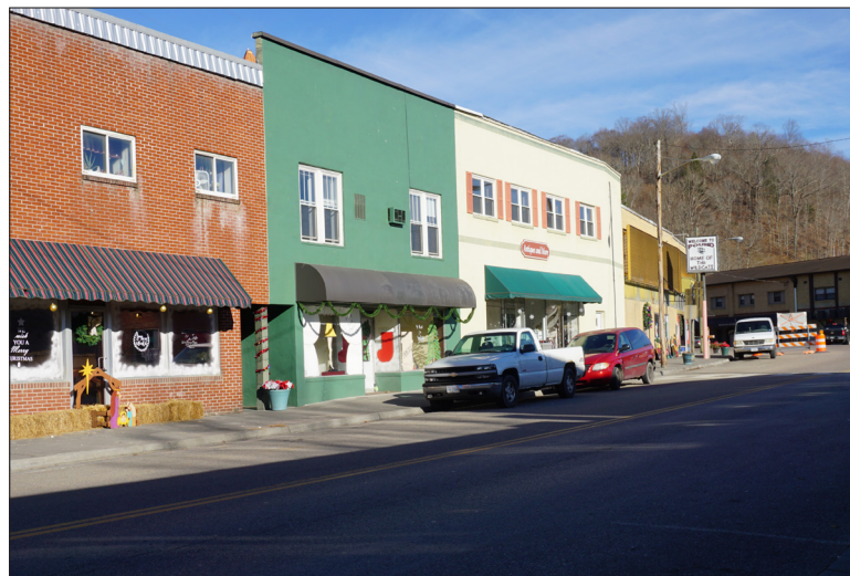
Diverse material/color approaches to downtown facade. Future retaining wall should be integrated with surrounding buildings.
