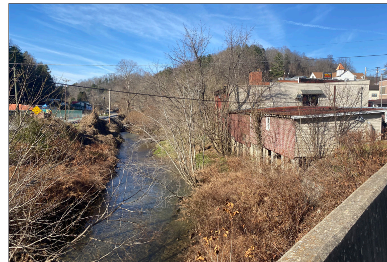
Crossing Pound River along Main Street (Rt. 23 Business). The bridge is walkable via a sidewalk.
