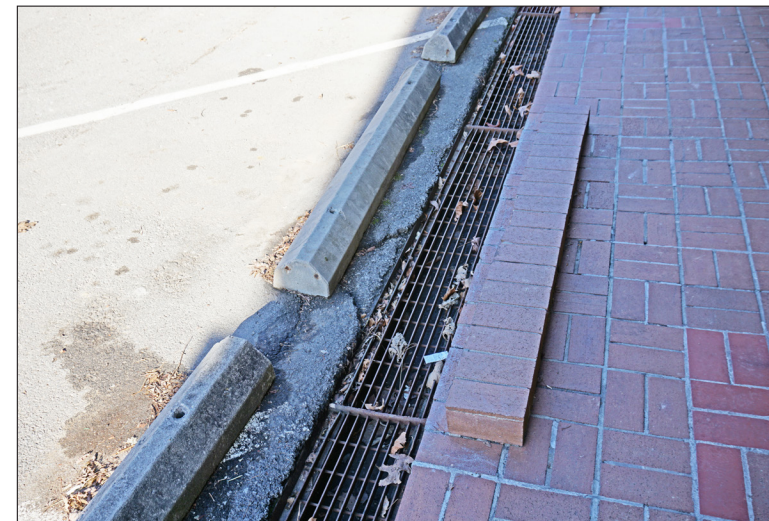
Brick paver sidewalk detail. Possible consideration for future sidewalk designs.
