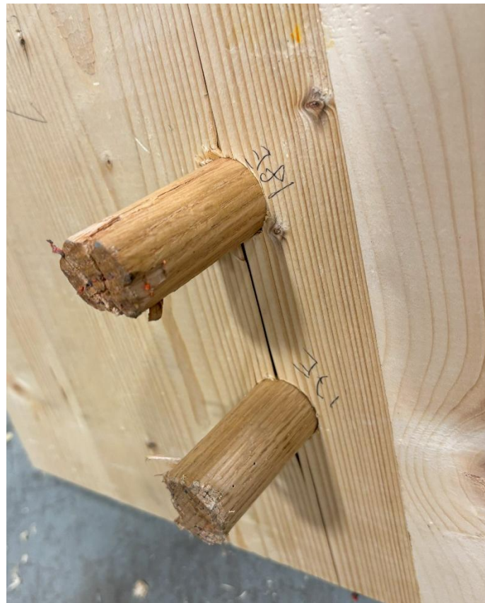
Figure 12: Splitting of Face Lamination and Peg Due to Undersized Holes
