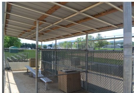
Northside High School, Roanoke, VA Example of a steel-fenced dugout with roof panel
