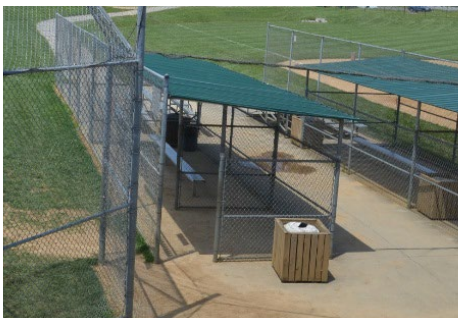
Northside High School, Roanoke, VA Example of a steel-fenced dugout with roof panel
