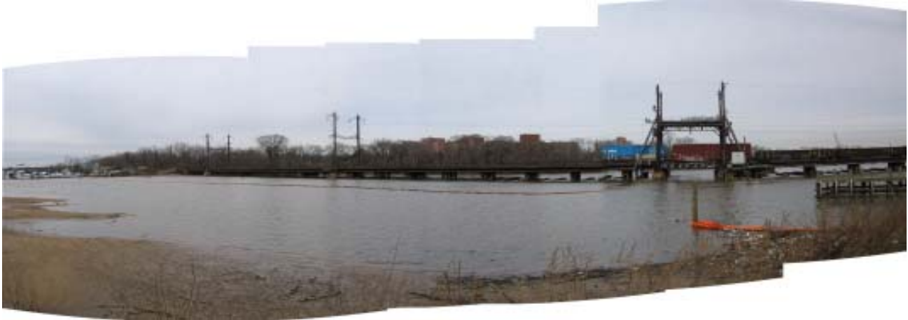
Figure 3-6 CSX Railway bridge, looking north
