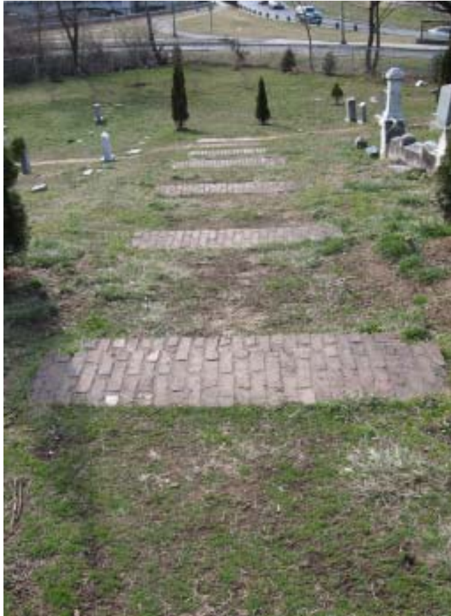
Figure 3-7 Brick earthwork steps, Congressional Cemetery, looking south
