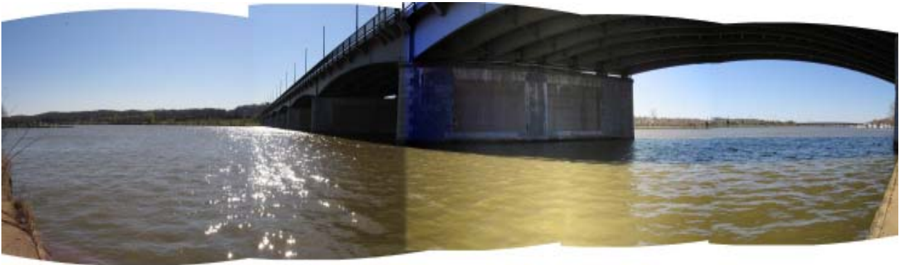
Figure 3-4 John Philip Sousa Bridge, looking south
