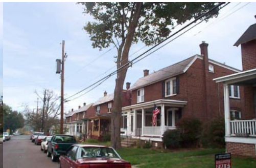
Existing Borough Housing
