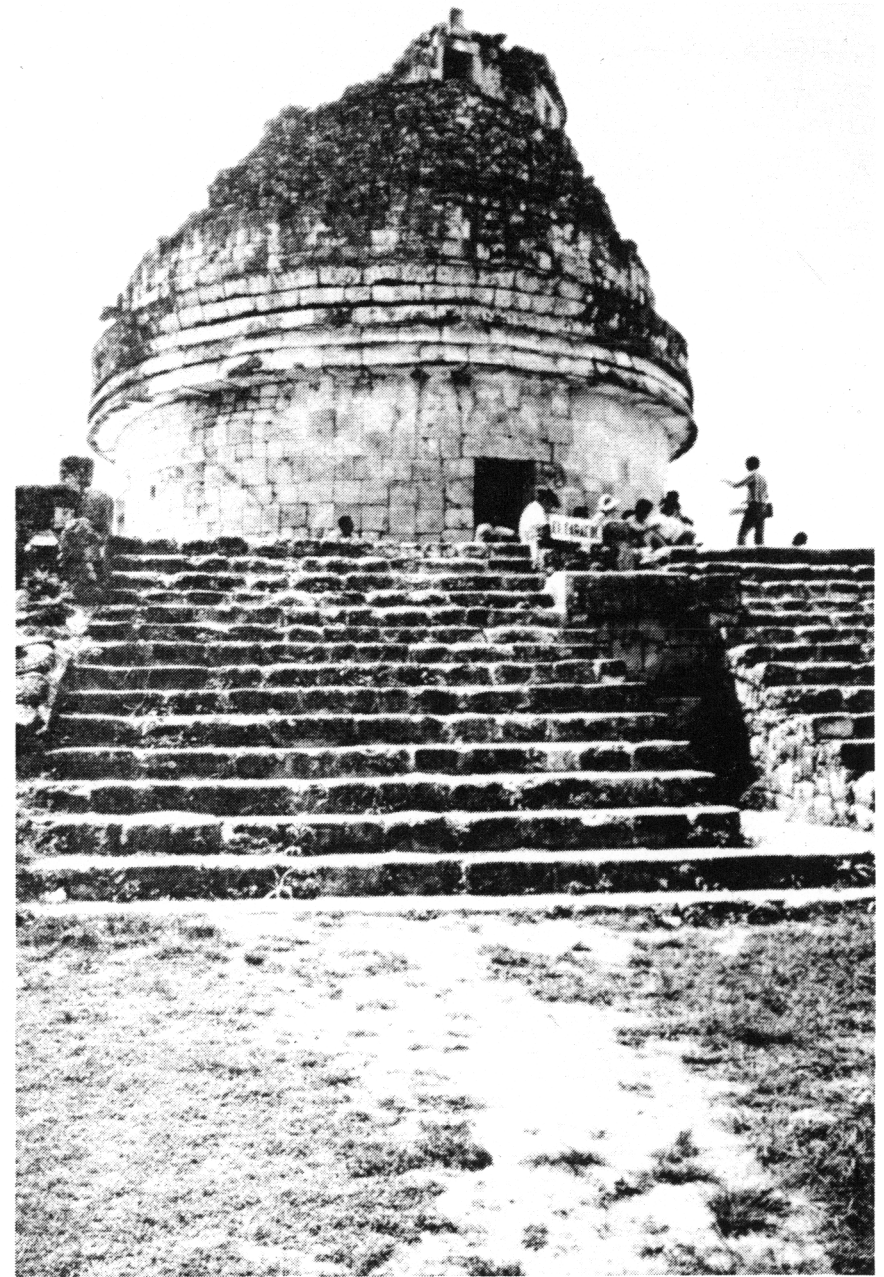
The Caracol at Chichén Itza, in Yucatan, included windows in its upper portion that could have been used for astronomical observation. (Robin Rector Krupp)
