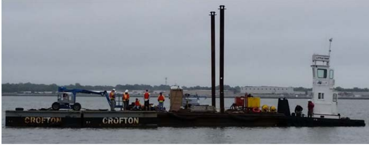
a) Tug Boat, Spud Barge, and Genie Lift
