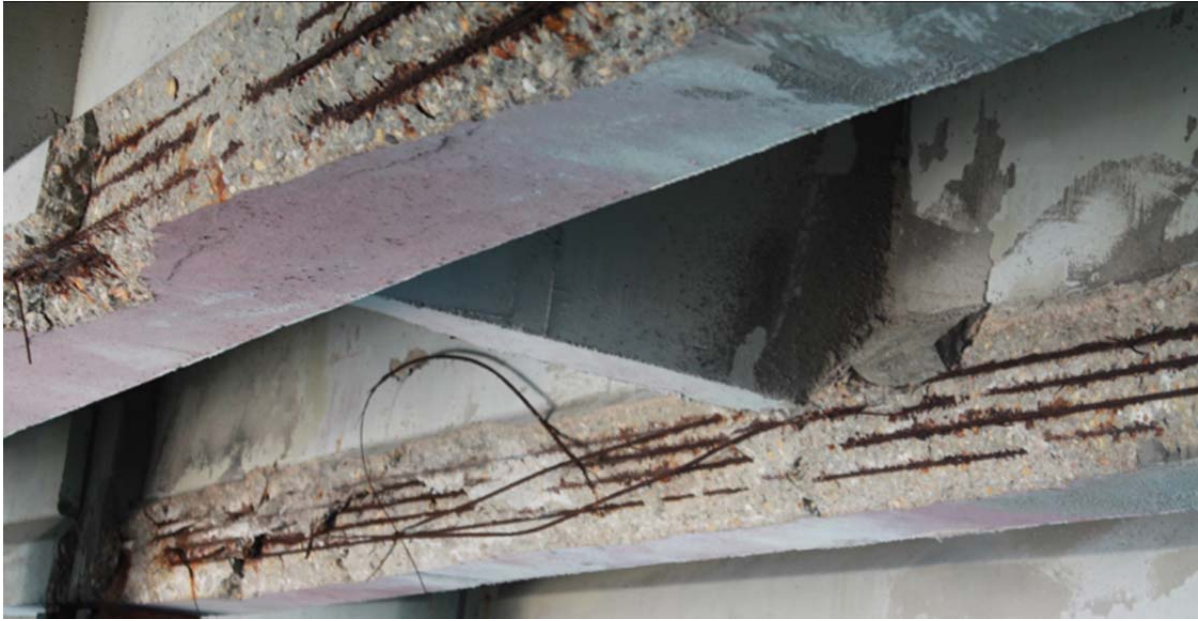
a) Girder 7 on left, Girder 8 on right
