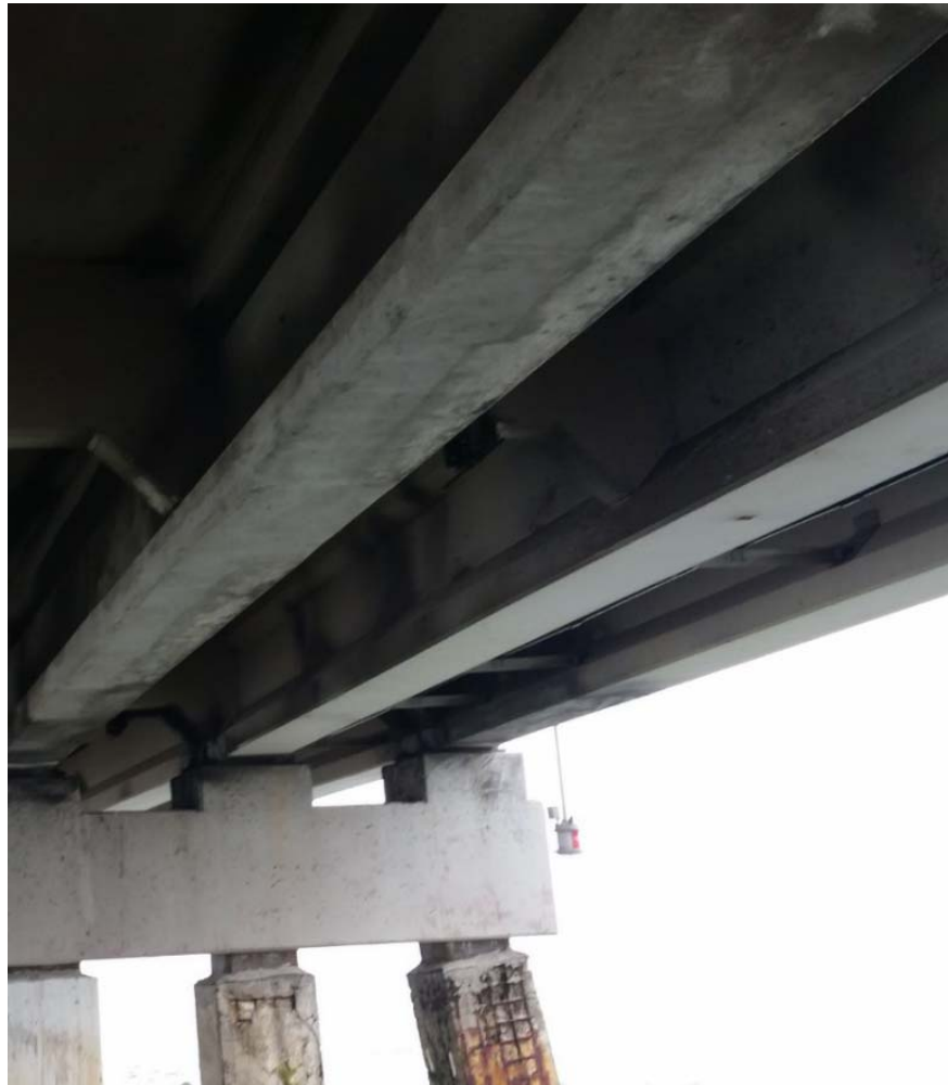
Figure 25: Shotcrete on Girder 5 Bottom Flange
