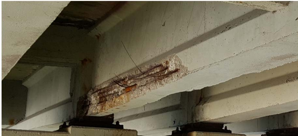
a) Girder 4 Bottom Flange at Support
