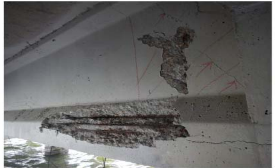
PHOTO K (BEAM 8, SPAN 31)
