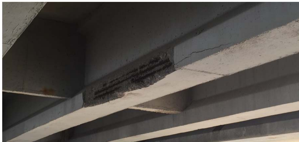
b) Midspan of Girder 4 Bottom Flange
