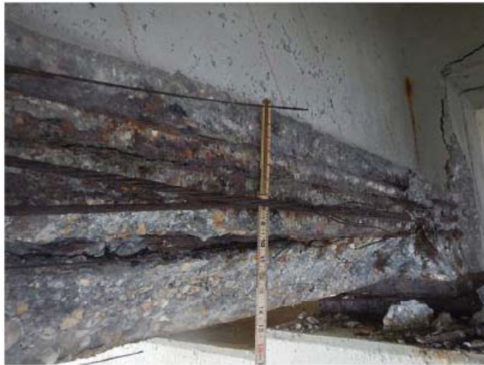
PHOTO O (BEAM 4, SPAN 34)
