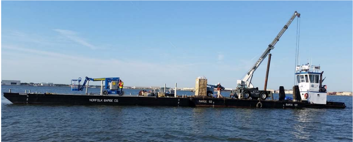
a) Float Barge, Spud Barge, Man Lift, Crane, Tug Boat
