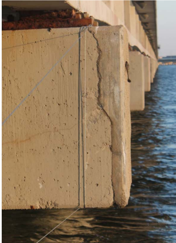
Figure 33: Chokers Wrapped Around Pier Cap
