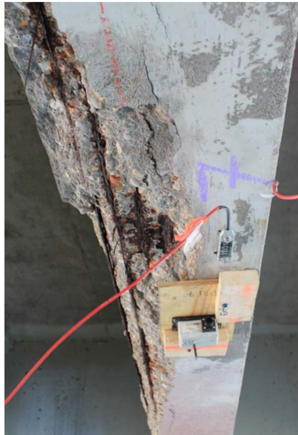
c) Girder 7 Midspan Soffit
