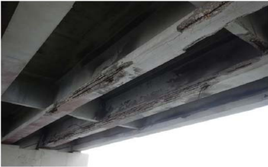
PHOTO H (BEAMS 7 & 8, SPAN 31)
