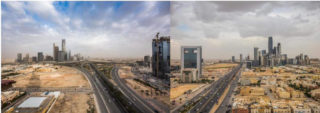
Figure 4. Aerial images show patches of vacant lands alongside major highways in Riyadh (alriyadh.com)
