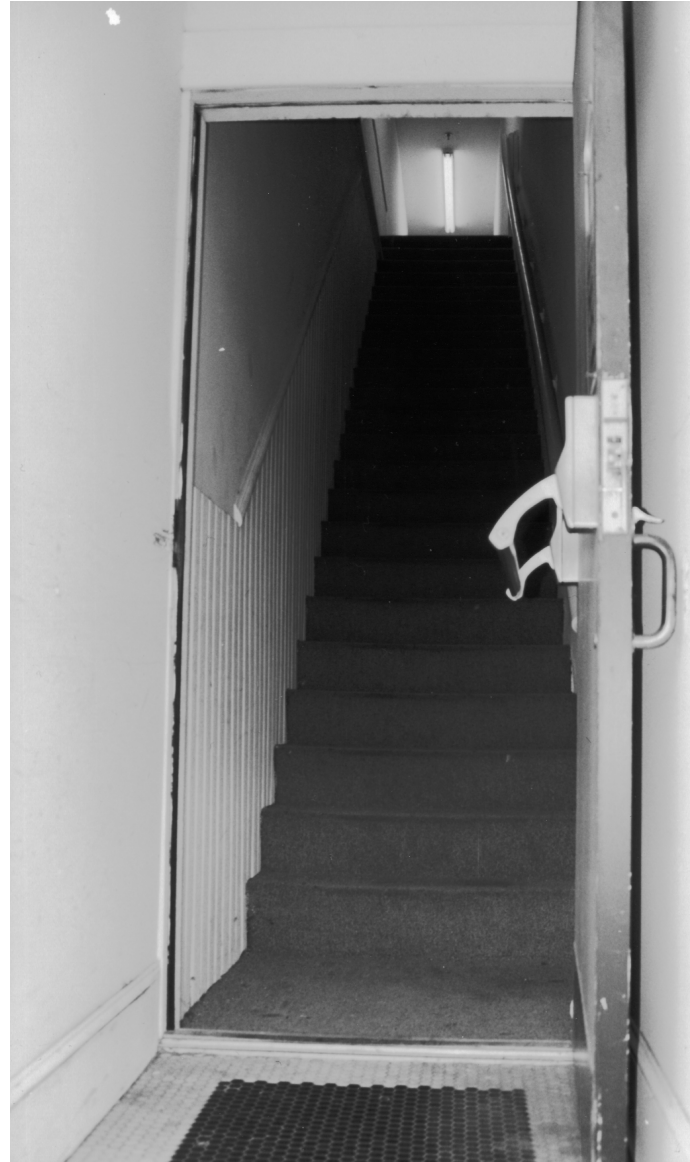
above: Typical entry stair along Salem Avenue; dark and narrow, with no visual connection to door at top of stair.
