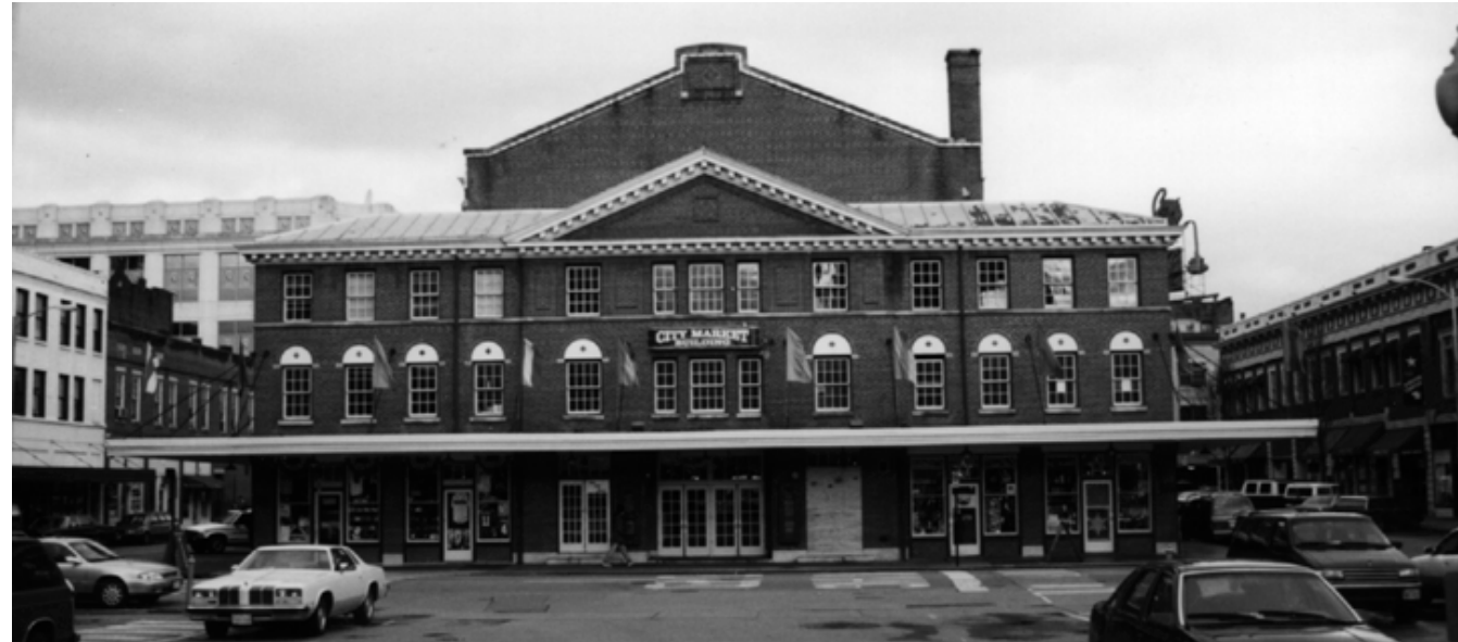
above: Front view of the City Market building.
