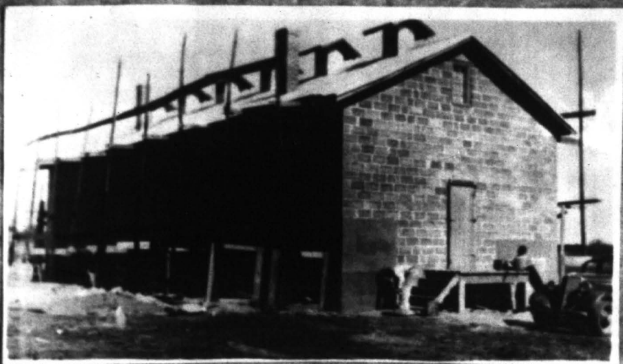
5,000 Bushel Storage House under Construction - Caroline County
