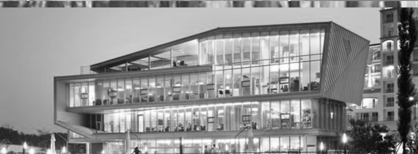
La-cubo Commercial Facility in the Republic of Korea by JUNGLIM Architecture
