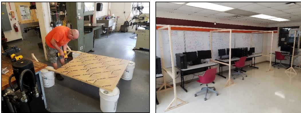
Figure 4 – Plexiglass partitions during construction (left), CAD lab partition placement (right).
