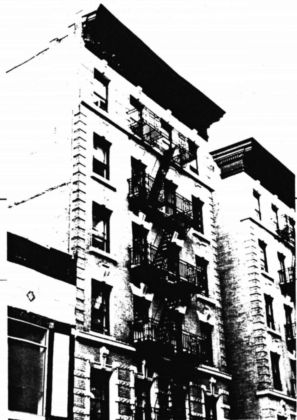
Typical New York tenement housing stock, holding the east end of the 103rd and Broadway site, on 103rd
