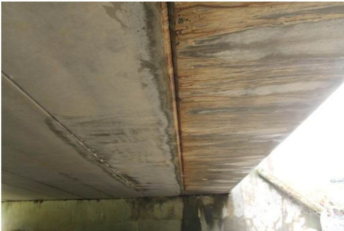
Figure 2. Leaking joint
