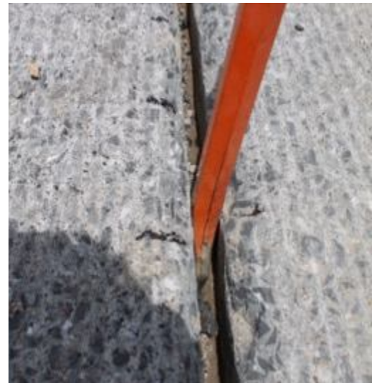
Figure 112. Removing grout from joints
