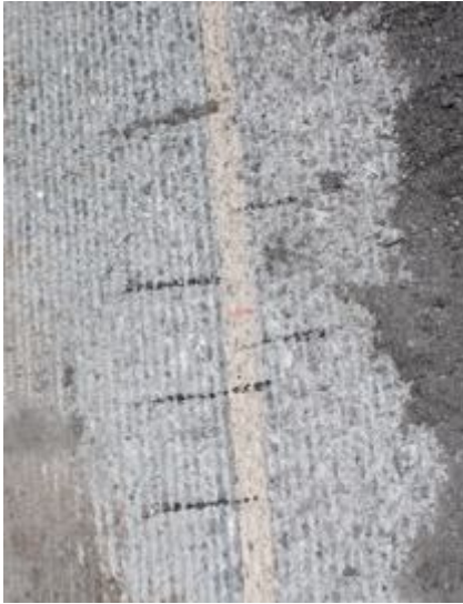
Figure 114. Reinforcing steel locations
