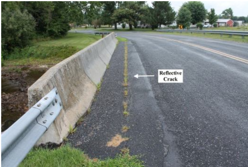
Figure 1. Reflective cracking
