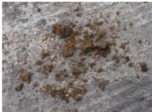
Figure 110. Deteriorated grout
