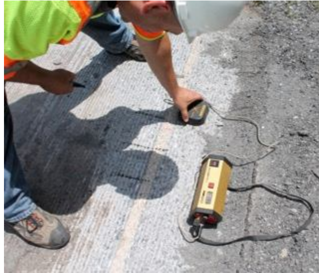
Figure 115. Locating steel with pachometer
