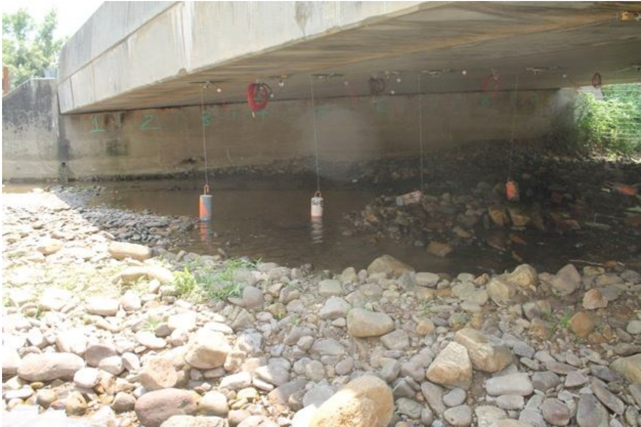
Figure 46. Deflectometers with weights attached
