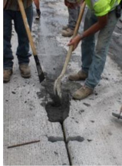
Figure 129. Spreading VHPC with shovels and scoops
