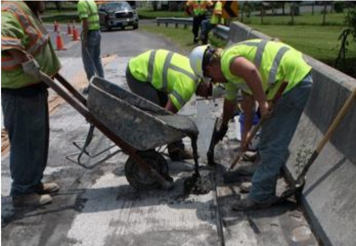
Figure 128. Dumping VHPC from wheelbarrow
