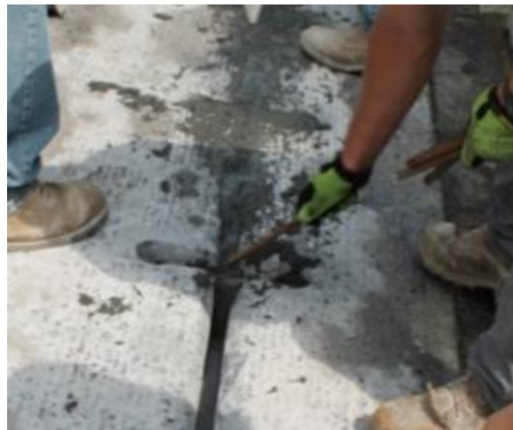
Figure 130. Placing reinforcing steel in dog bones
