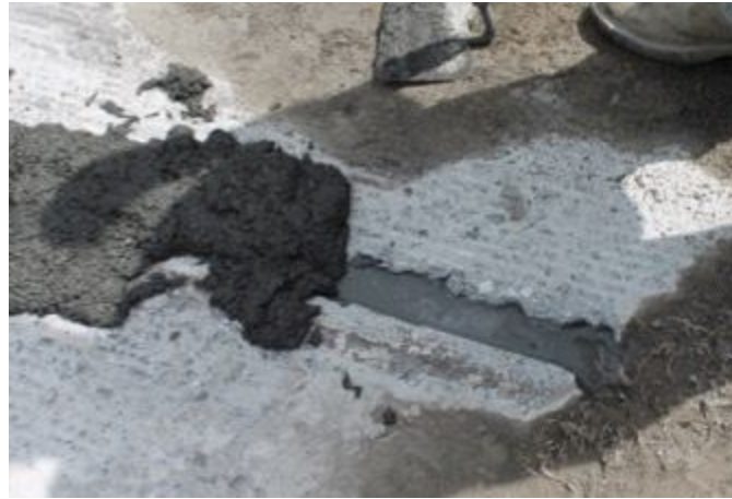
Figure 133. Water building up at the end of joint
