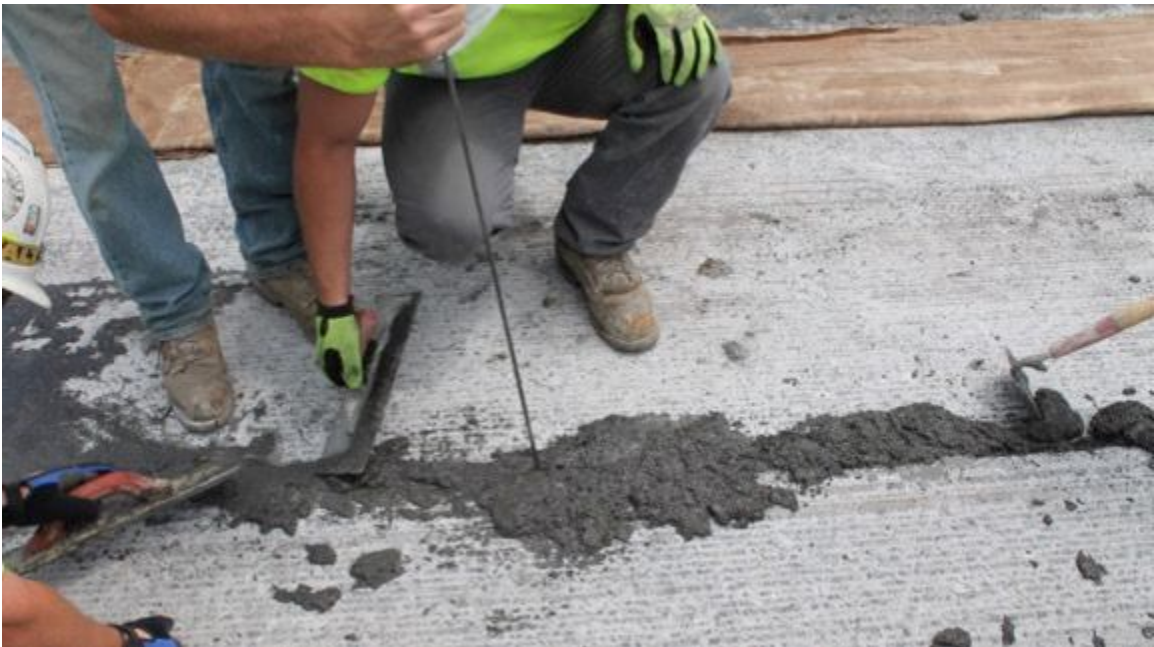
Figure 132. Rodding VHPC where batches meet
