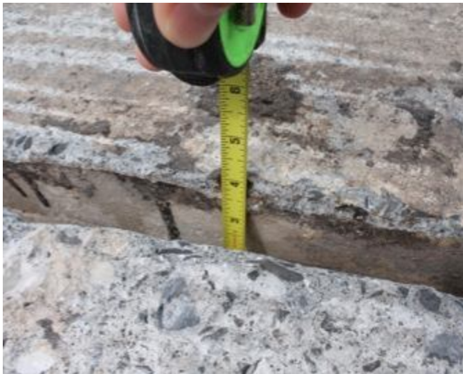
Figure 111. Typical depth of cleared joints
