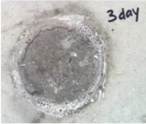
Figure 77. Typical VHPC 2 day to 5 day failure
