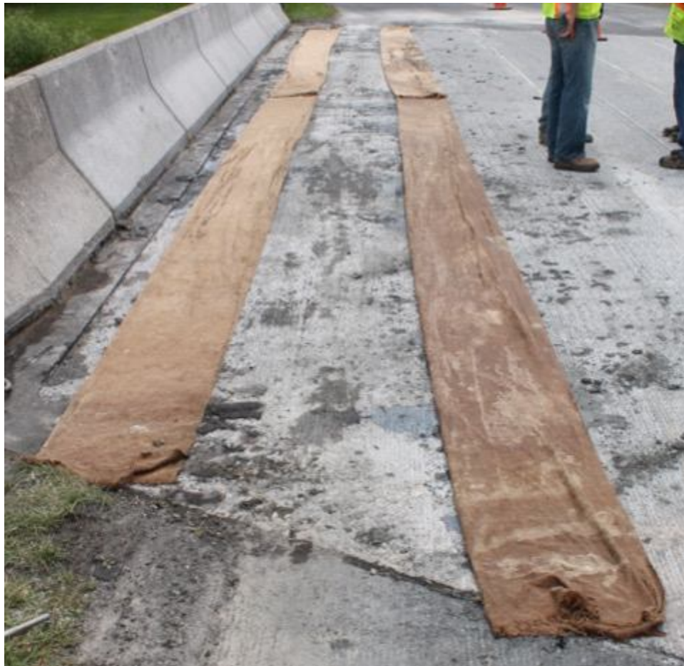
Figure 136. Wet burlap covered joints
