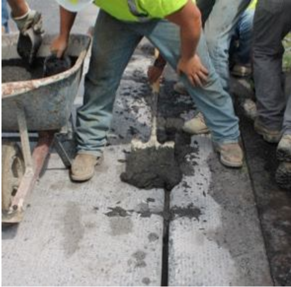
Figure 129. Spreading VHPC with shovels and scoops
