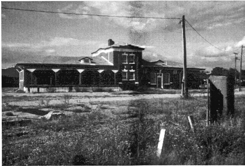
ATLANTIC COAST LINE PASSENGER STATION, TARBORO: 1994 THE ABANDONED EAST-WEST RAILROAD LINE RUNS ON THE STATION'S OPPOSITE SIDE
