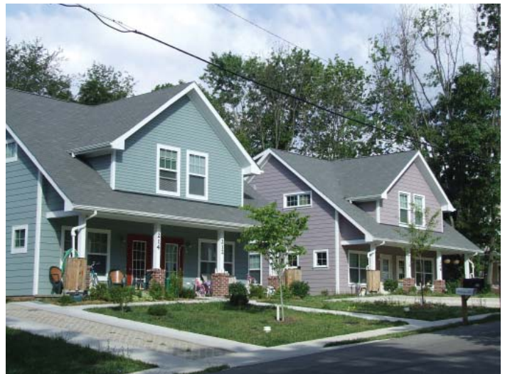
Example of a desirable high density residential development. Note how each residence addresses the street and has a single front entry.
