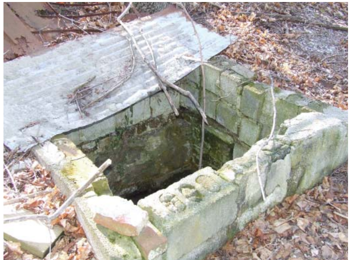
Old spring box found near the intersection of Clay and Penn Streets.
