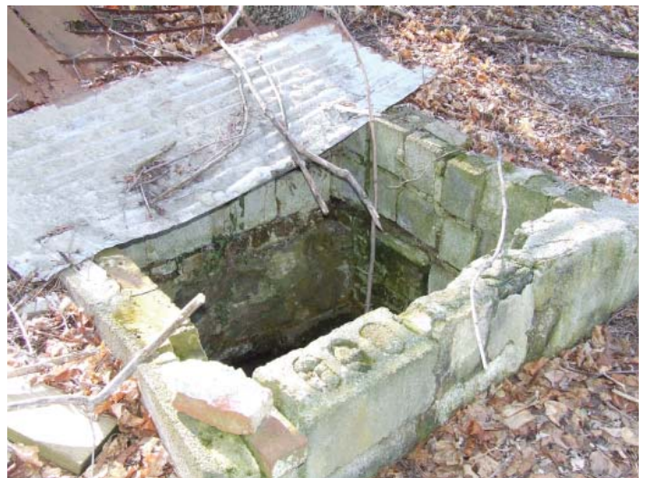
Spring box located just off of Penn Street, adjacent to a gravel alley between Clay and Washington Streets.
