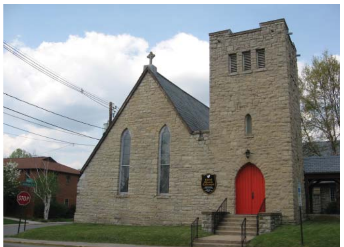
Christ Episcopal Church located on the corner of Church Street and Jackson Street. The earliest portion of the church was built in 1879.
