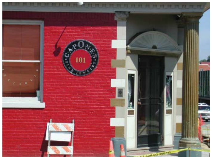
Historic: Corner condition at the junction of Roanoke Street and Main Street.
