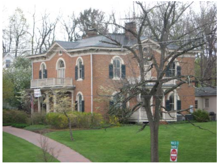
The Thomas Conner House faces a T-intersection at Draper Street and Lee Street.
