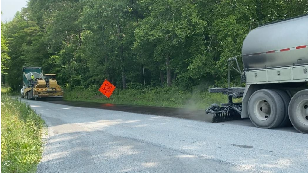
Figure 7. Chip Spreader following asphalt distributor
