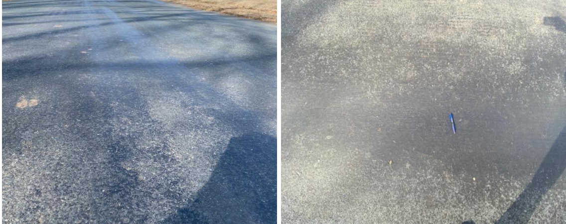
Figure 20. Flushing at the end of the route
