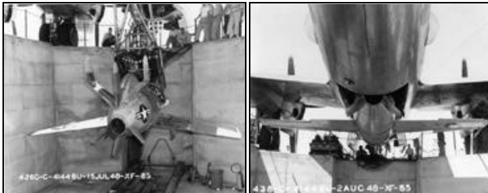
Figure 1.16: (left) The Goblin Being Retracted in to the belly of the B-29, Monstro, and (right) Fully Retracted [2].
