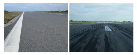
(a) Surface area generally in good condition (b) Localised rubber deposits Figure 4 - Surface Appearance after 3 years in Service
