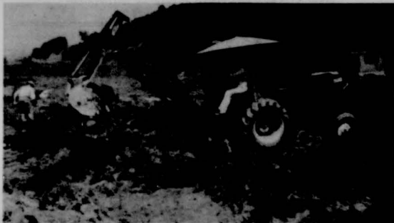
Digging Open Drain Ditch On Buhrman Farm Botetourt County
