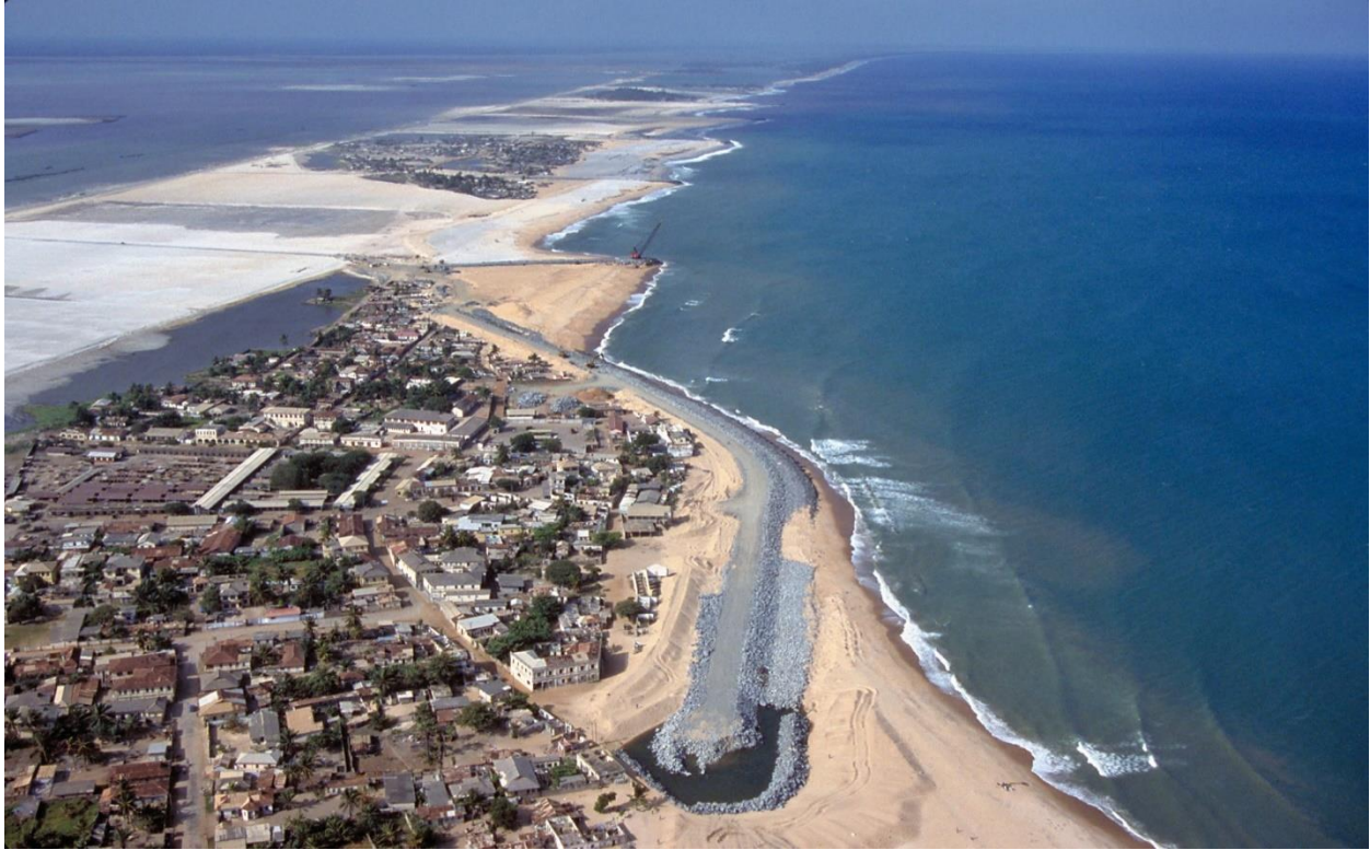
Figure 1.6: An Aerial photograph of the Keta Sea Defense Works Project (KSDW) adopted from Research Planning Inc.
