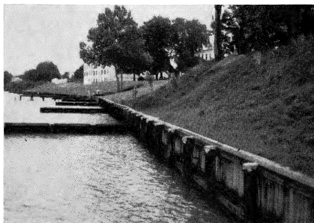
An example of effective erosion control which can be achieved with properly engineered structures, bank sloping, and vegetation.
