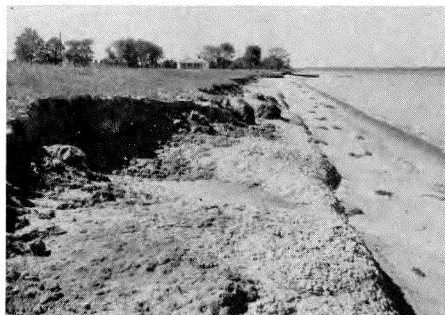
An unsuccessful attempt by the landowner to control bank erosion by sloping and reseeded. Most of this damage was done by a single storm.
