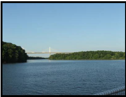
James River near Interstate-295 bridge, June 2007.
