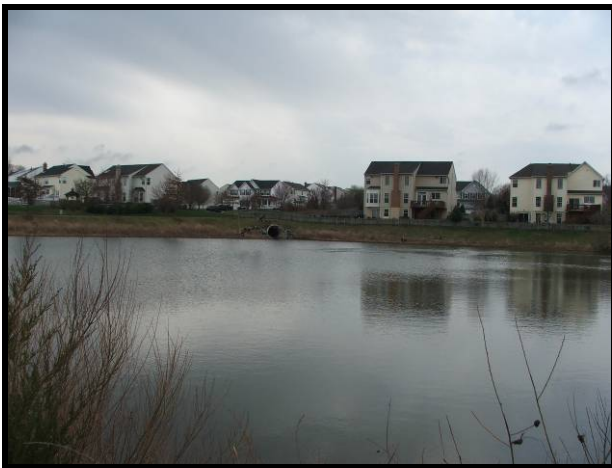
Stormwater pond for a residential development in Leesburg, Va., March 2008.
