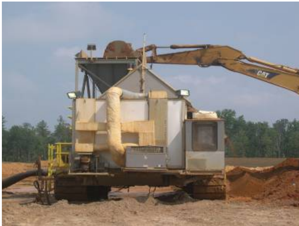
Figure 5. Mobile mining unit receiving ore. The ore is crushed and coarse-screened here and then pumped to the wet mill for processing. Photo courtesy of Chuck Stilson/Iluka.
