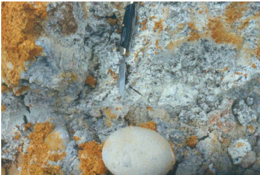
Figure 11. Granitic saprolite with Coastal Plain cobbles and weathered soil above. This photo is from an exploration well in the northern portion of Old Hickory. Saprolites like this one underlie the mineral sands deposits at depth ranging from < 5 to > 10 m. Photo courtesy of W. L. Daniels.
