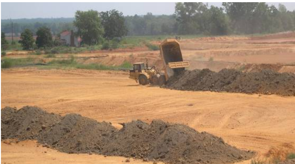
Figure 15. Topsoil being returned to re-graded mining pit. The topsoil will be graded out to nominal 15 cm thickness with a bulldozer. Photo courtesy of Chuck Stilson/Iluka.
