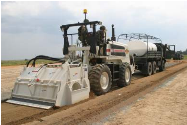
Figure 2-1. A pulverizer mixing stabilizers into the soil. (Newman 2005)
