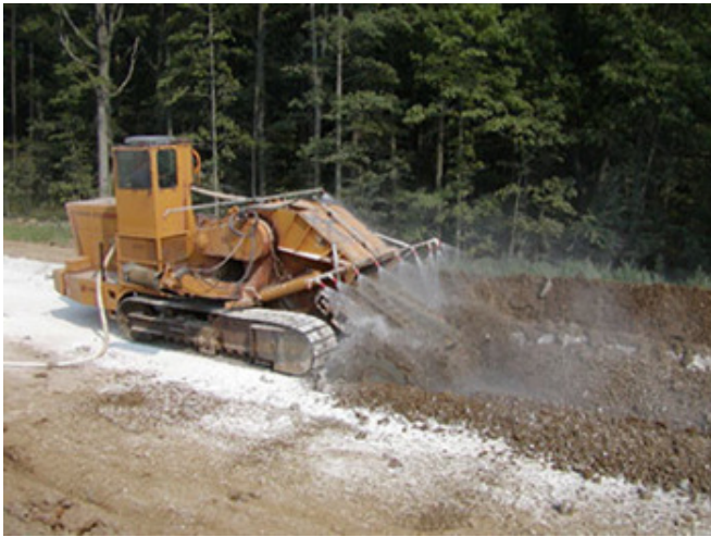
Figure 7-1. J. H. Becker Company (2006) equipment mixing lime into soil.
