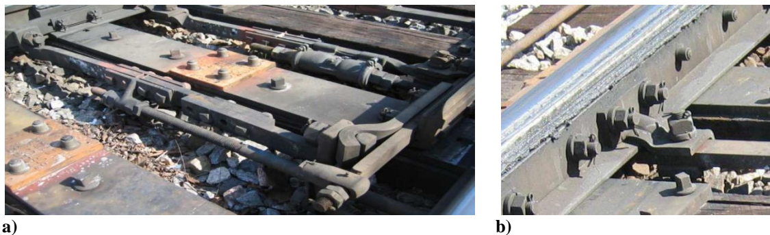
Figure 3.3. Snapshots of a) a lock rod and b) its clip
