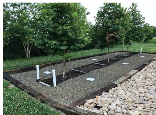
Figure 3. Gravel bed bioretention system in June 2021, one year after construction and tree planting.
