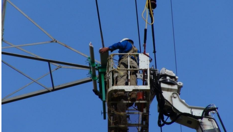
Figure 2.5 DSR Installation on TVA 161 kV Line
