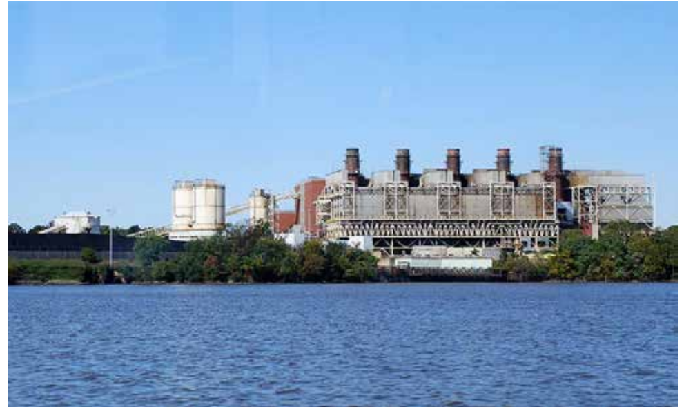
Fig. 10: Photograph of the Alexandria Power Plant while still in operation from across the Potomac River
