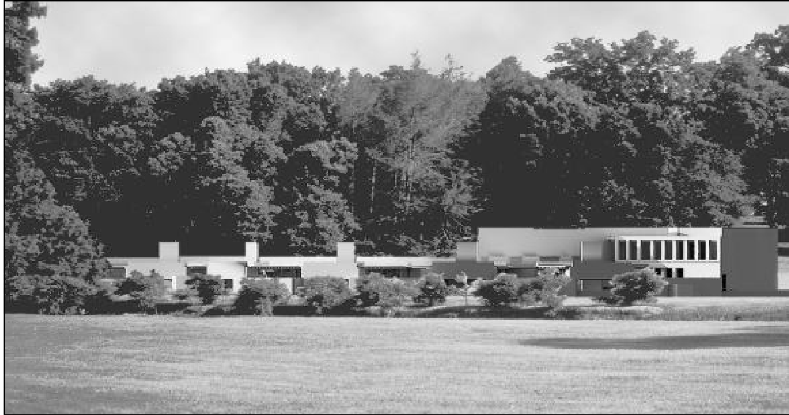
Northern elevation on Site
