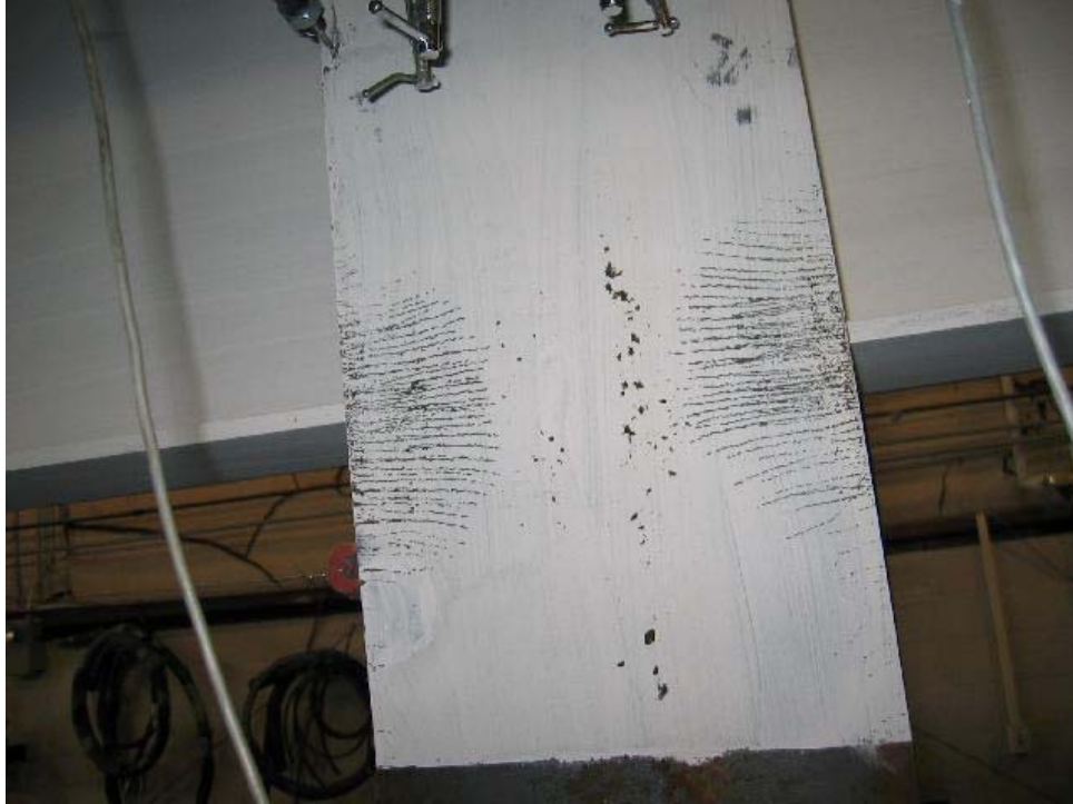
FIGURE 3.11: WHITEWASH FLAKING ON SOUTH COLUMN FLANGE AFTER COMPLETION OF LOAD SEQUENCE #5
