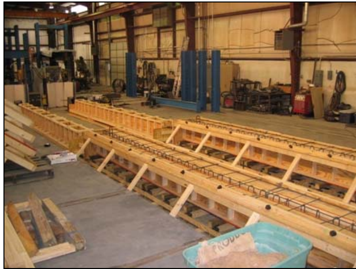
Figure 2. Prestressing bed.
