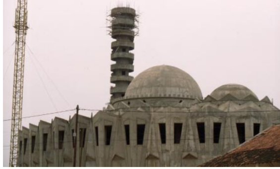
Mosque Under Construction
