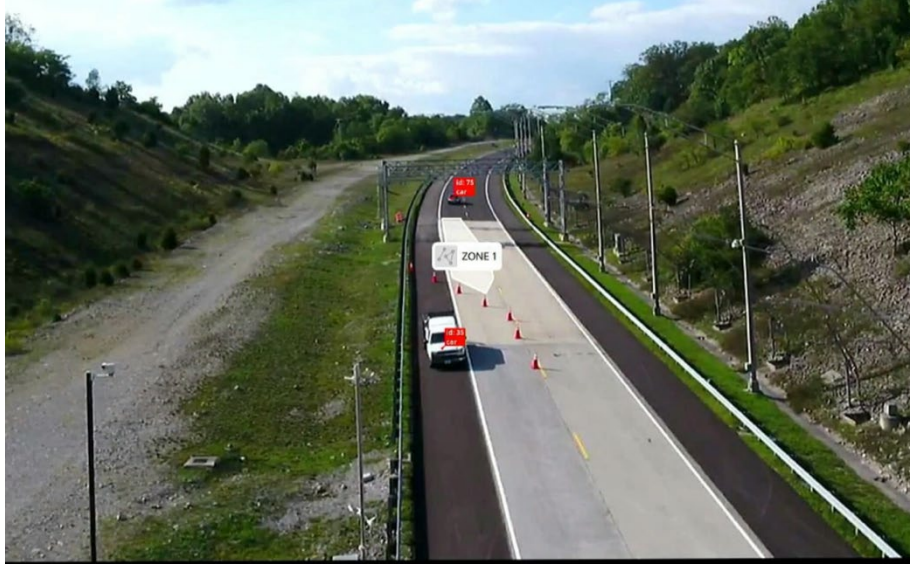
Figure 8. Photo. Drone video view of work zone.
