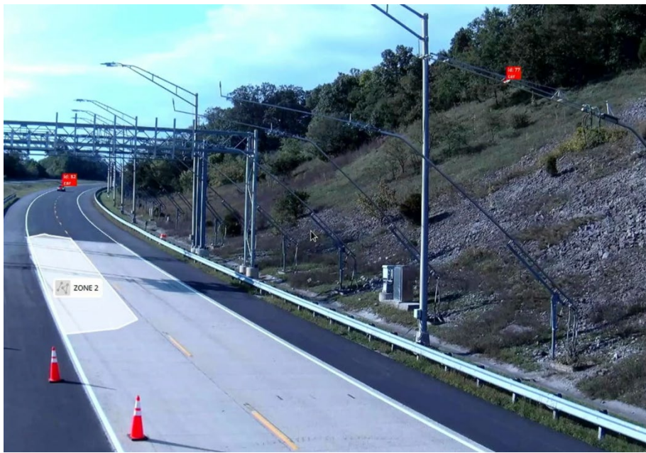
Figure 9. Photo. Telescoping pole-mounted camera view of work zone.
