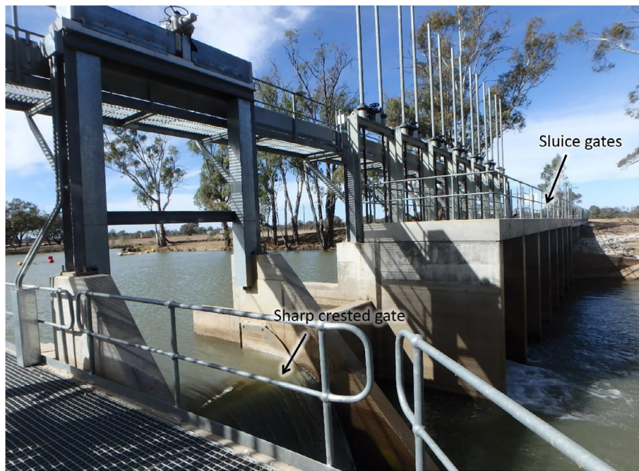
Fig. 2. Colligen Creek Weir with one overshot weir (left) and seven undershot weirs (right). The fishway is located to the left of the overshot weir.
