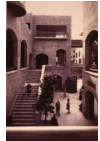
after renovation, shops and restaurants connected by network of open-air circulation (42)
