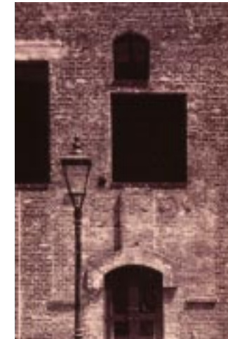
brick wall during use as warehouse (41)
