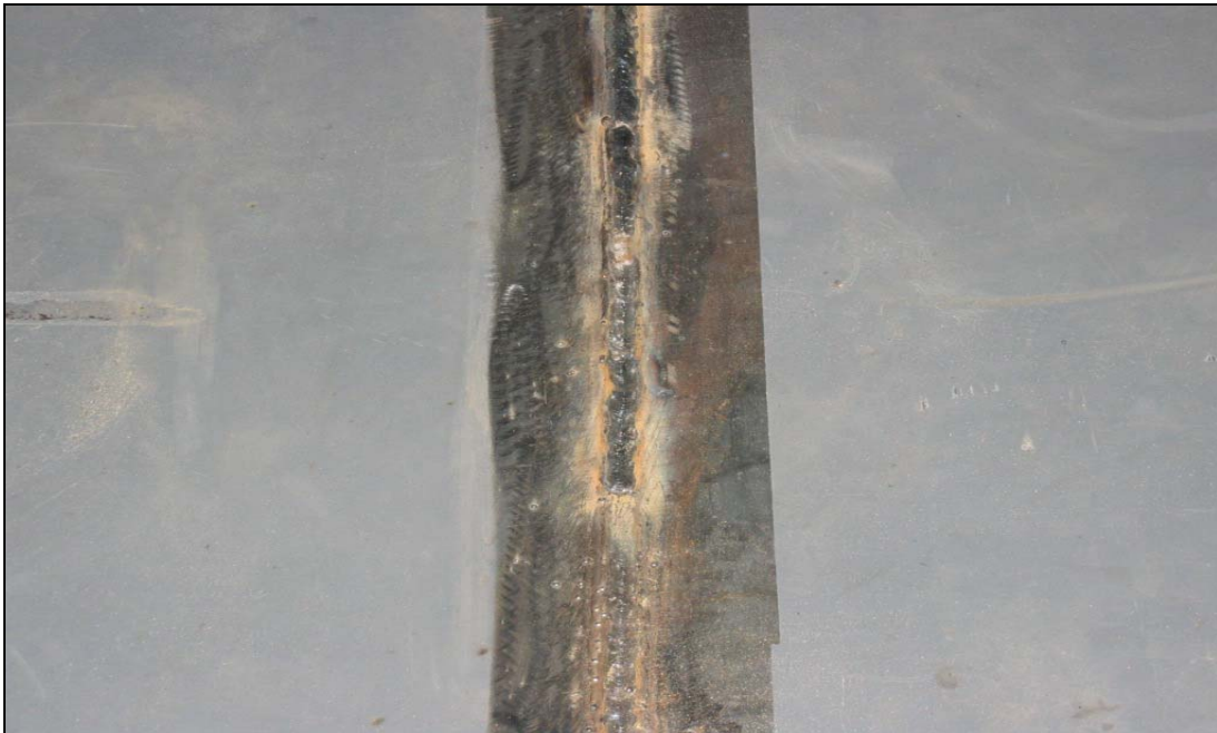
FIGURE 4.32: WELD SURFACE AT JOINT 3
