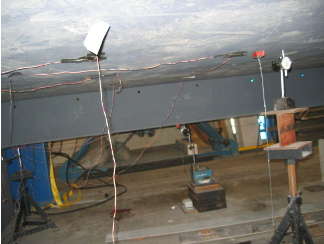
FIGURE 2.14: BOTTOM STEEL PLATE AT LOCATION OF MAXIMUM DEFLECTION
