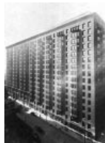
Notice the window depths in the load bearing walls of the Monadnock Building in Chicago. The walls vary from 18 inches at the top to 6 feet at the base.
