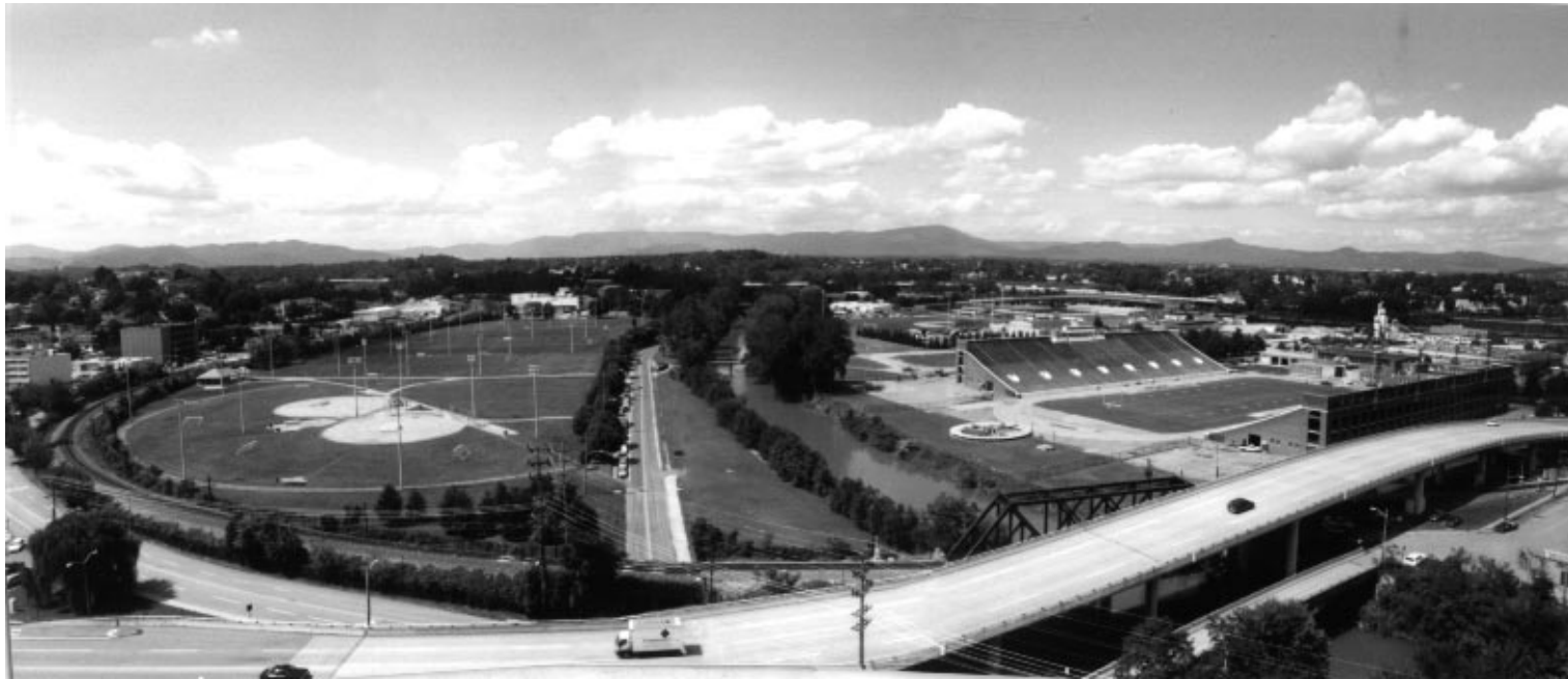
Looking west over the River's Edge Sports Complex from Roanoke Memorial Hospital
