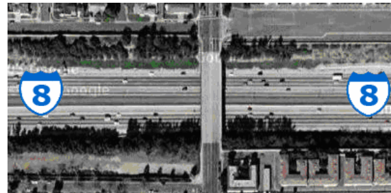
Example of a highway 8 underpass
