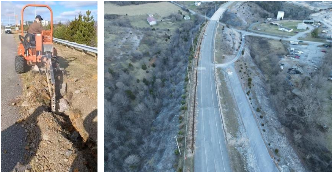
Figure 6. Photos. Virginia Smart Roads fiber optic trenching activities.
