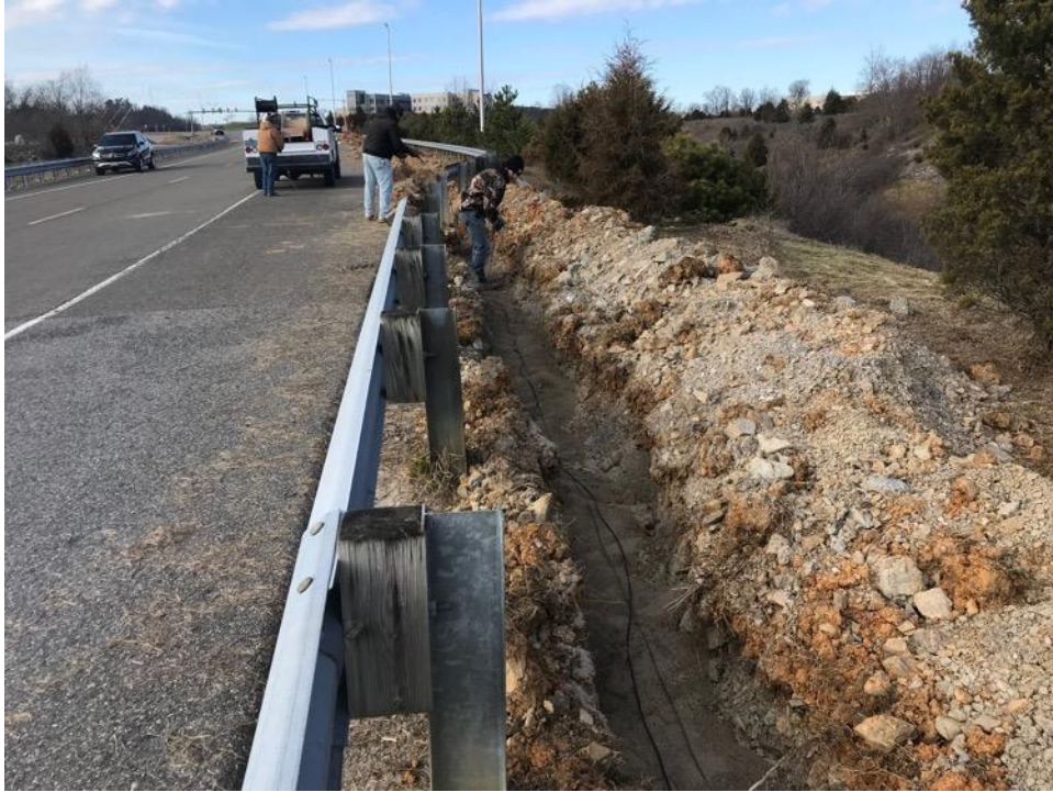
Figure 7. Photo. Virginia Smart Roads fiber optic laying activities.
