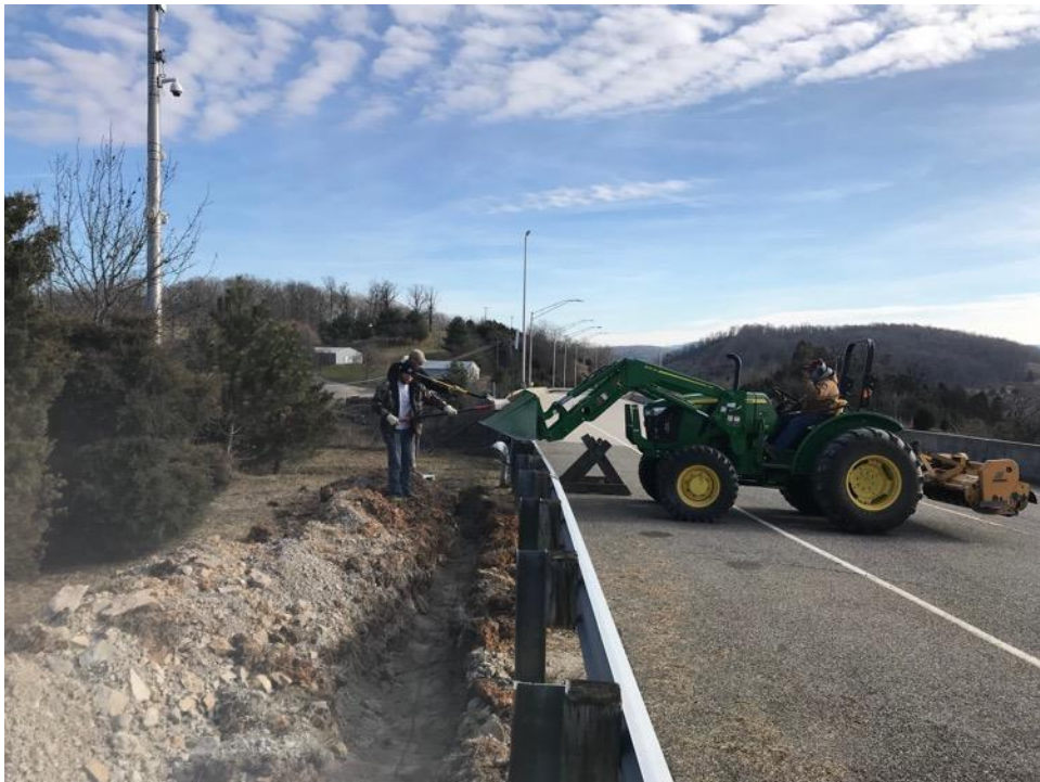
Figure 8. Photo. Virginia Smart Roads fiber optic backfilling activities.
