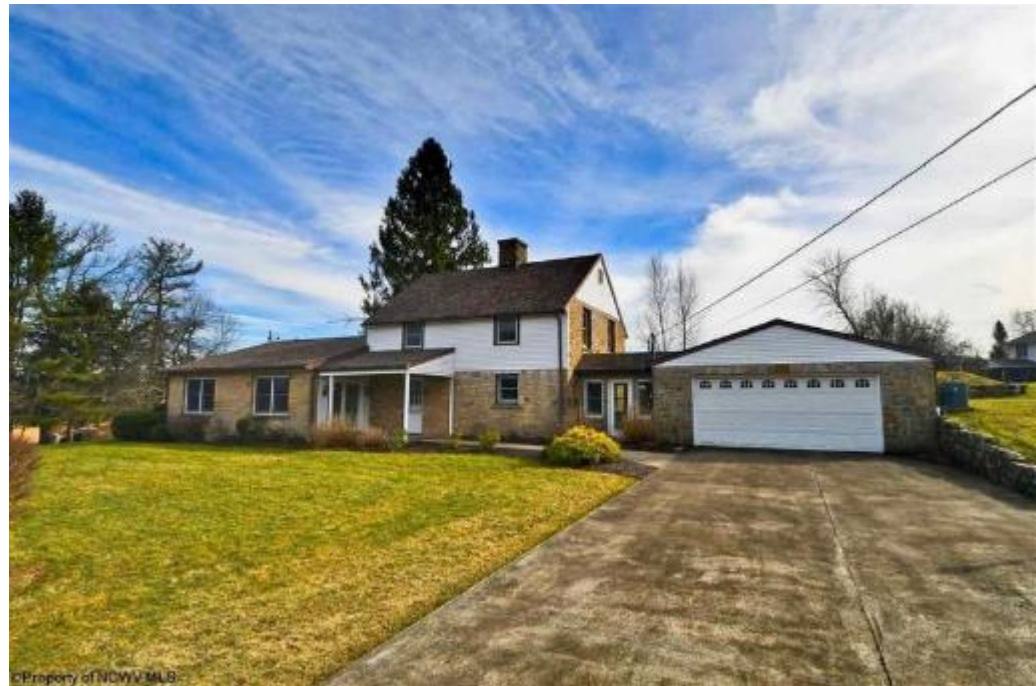
Renovated original house at Arthurdale
