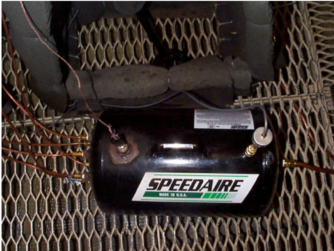
Figure 3.8: TEB Supply Air Plenum
