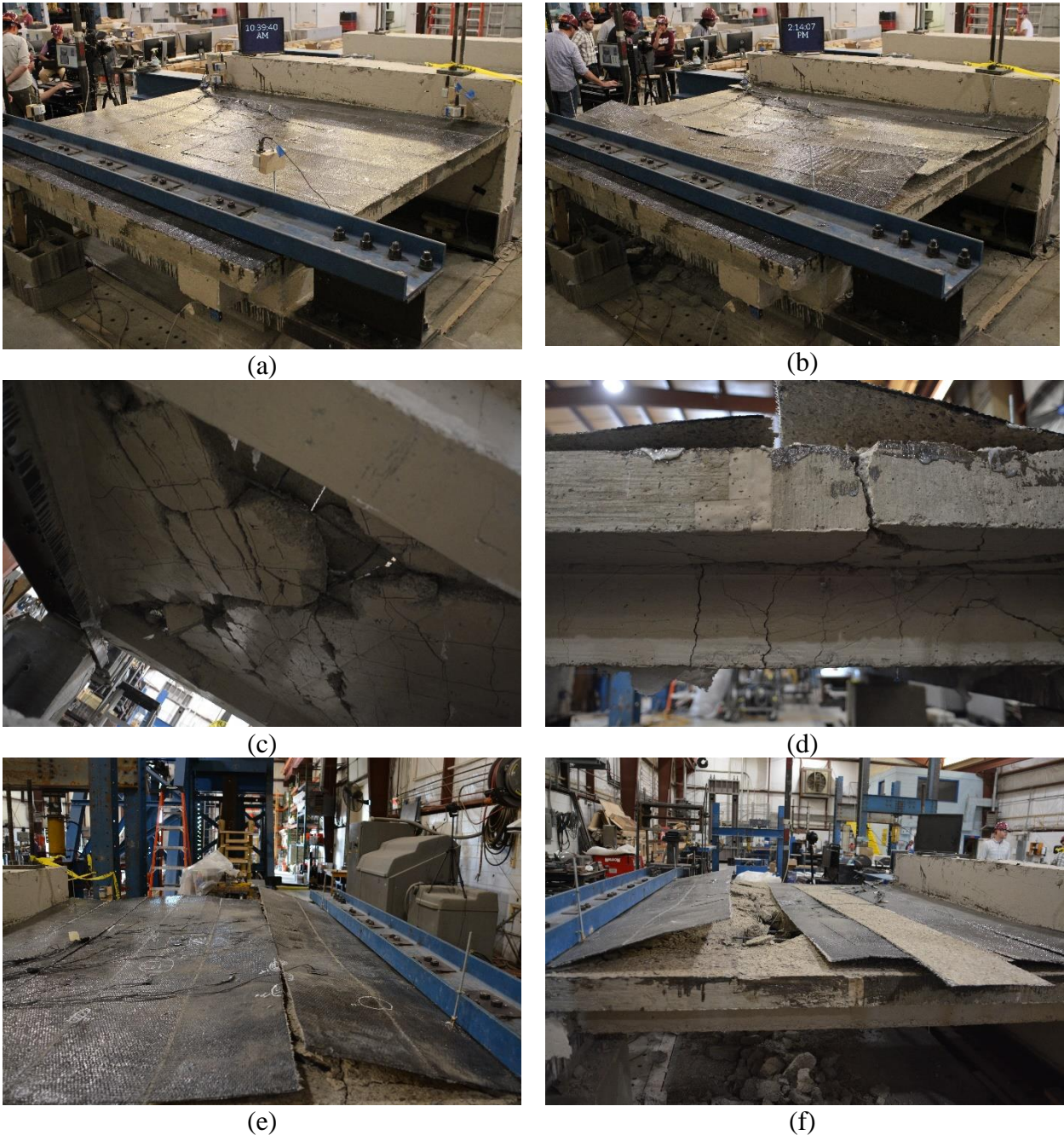
Figure 4-6. Photographs of Specimen CD8: a) Before Testing; b) Post-test Condition of the Specimen; c) Diagonal Tension Cracks and Section Loss in Concrete; d) Cracks in Chord Beam; e) FRP Debonding Near the Actuator; f) Spalling of Concrete Due after FRP Debonding.
